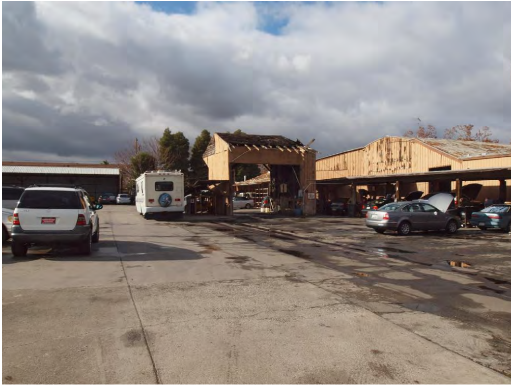
Rear of building, viewed facing west.
