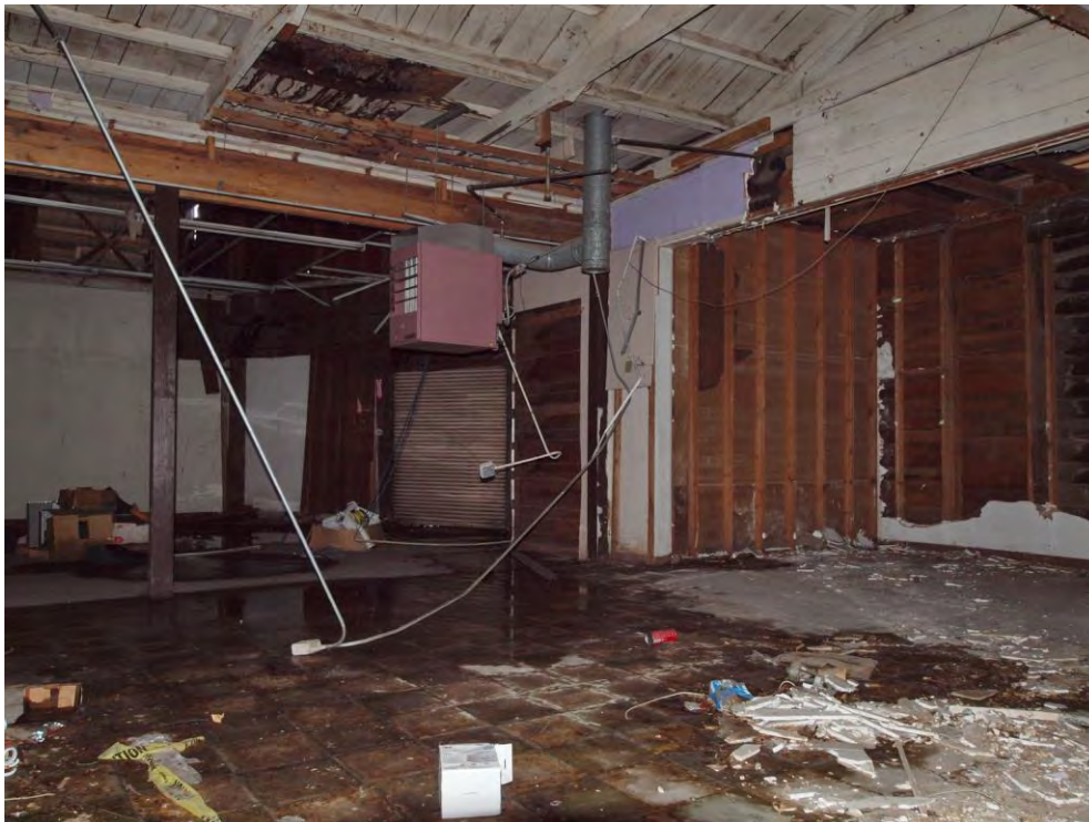
Rear addition area, viewed facing southeast.
