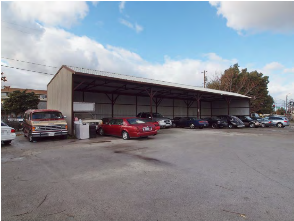
Open shed at west end of site, viewed facing northwest.
