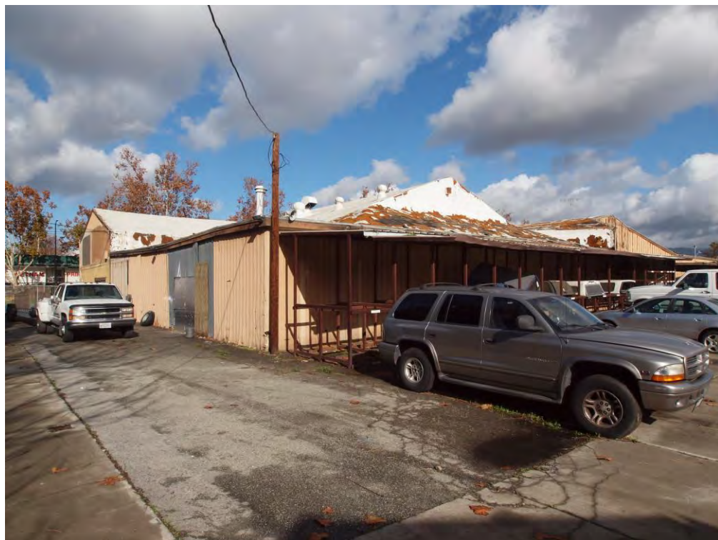
Southwest corner of building at rear, viewed facing northeast.
