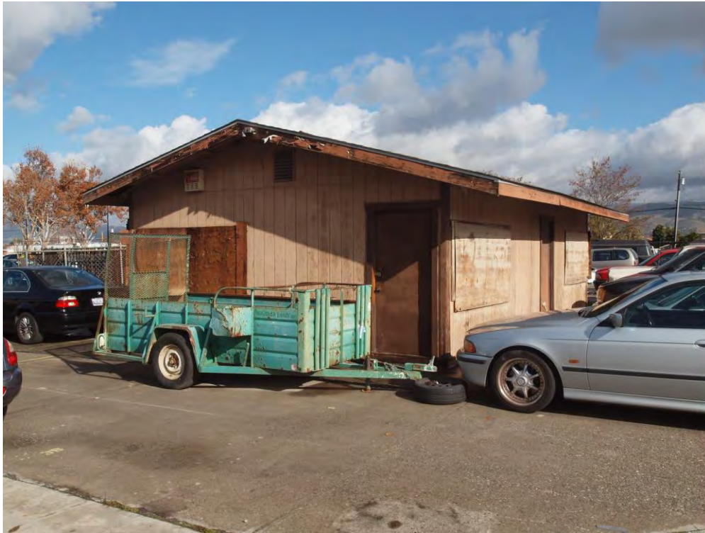
Ancillary structure at rear of car lot, viewed facing northeast.
