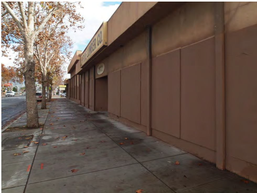
Front façade at East Santa Clara Street, viewed facing east.
