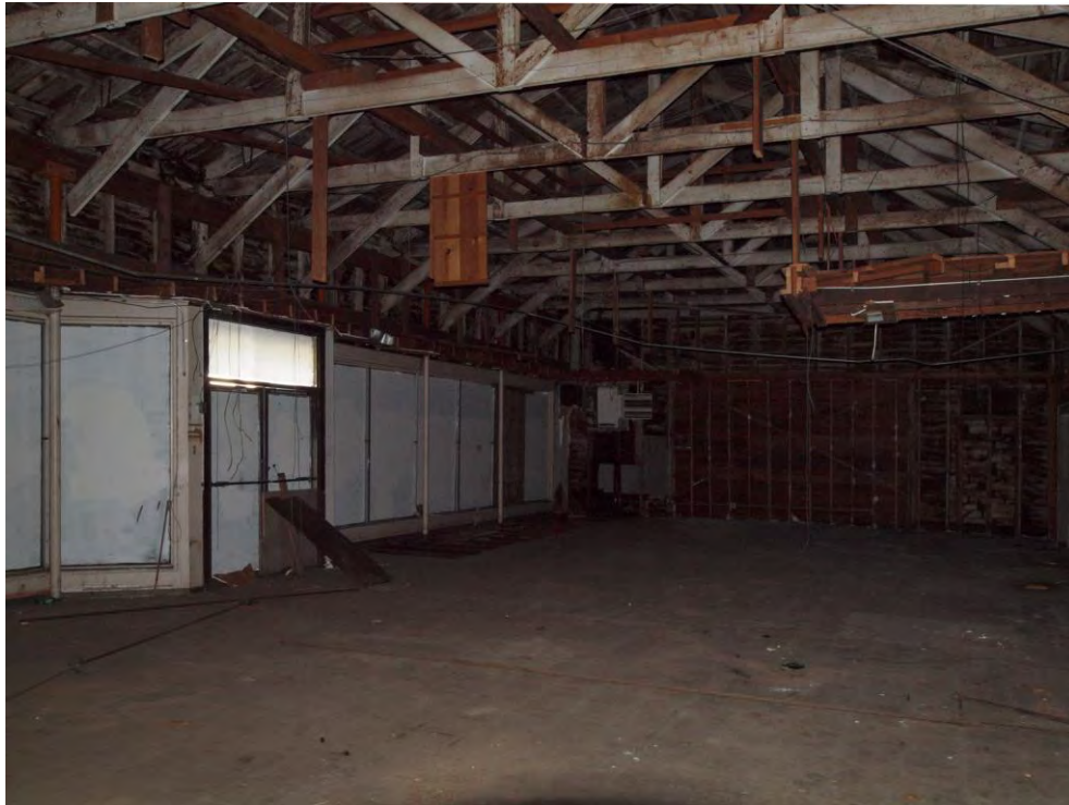
Interior of original mill area (later hardware store), viewed facing northeast.
