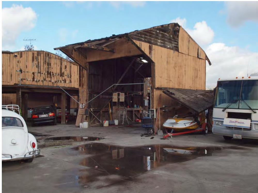
Drive-through, viewed facing northeast.
