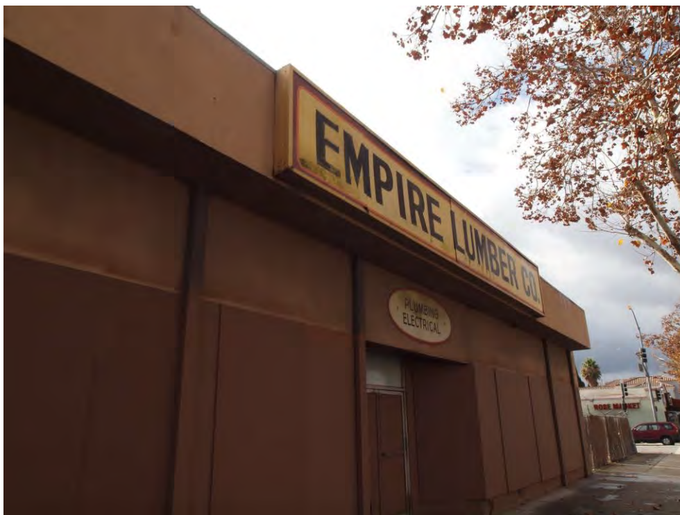
Detail view of front façade at boarded-up entry to hardware store area of Empire Lumber Co., viewed facing southwest.
