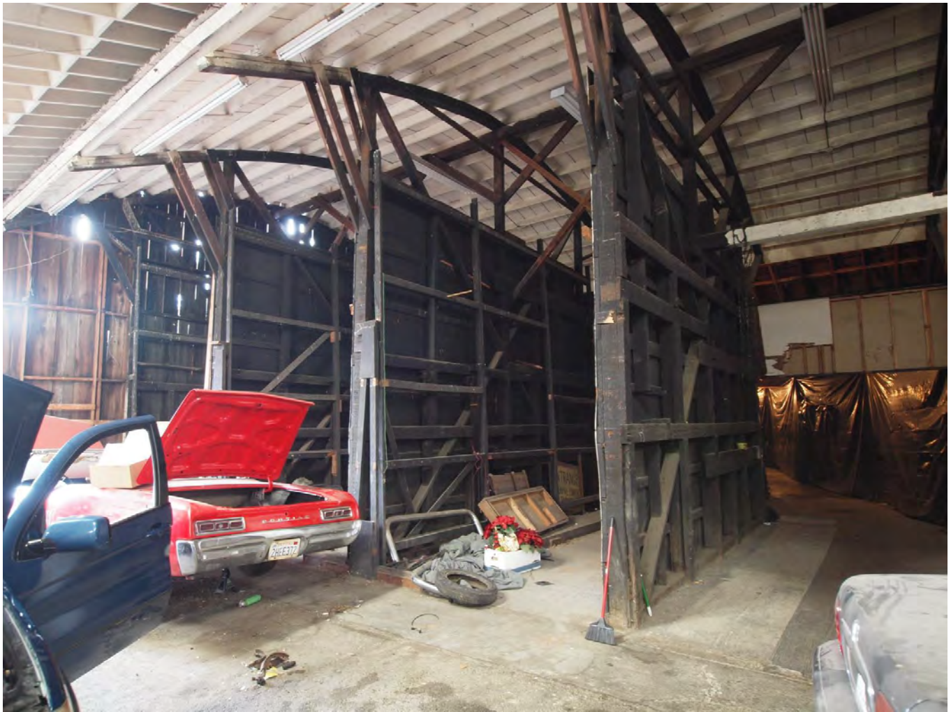
Original lumber store area, viewed facing southwest.
