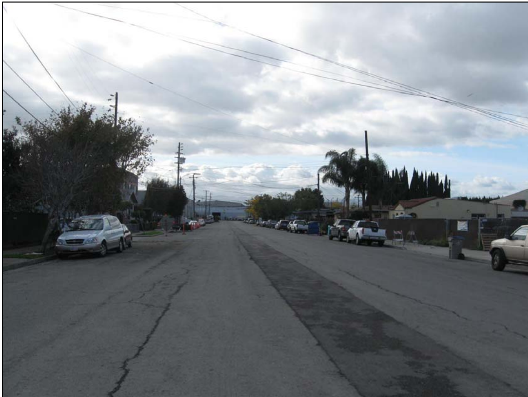
Photograph 9: Horning Street in front of the project site, facing west
