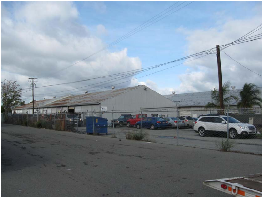
Photograph 3: View into the project site from the 13 th Street remnant, facing northeast
