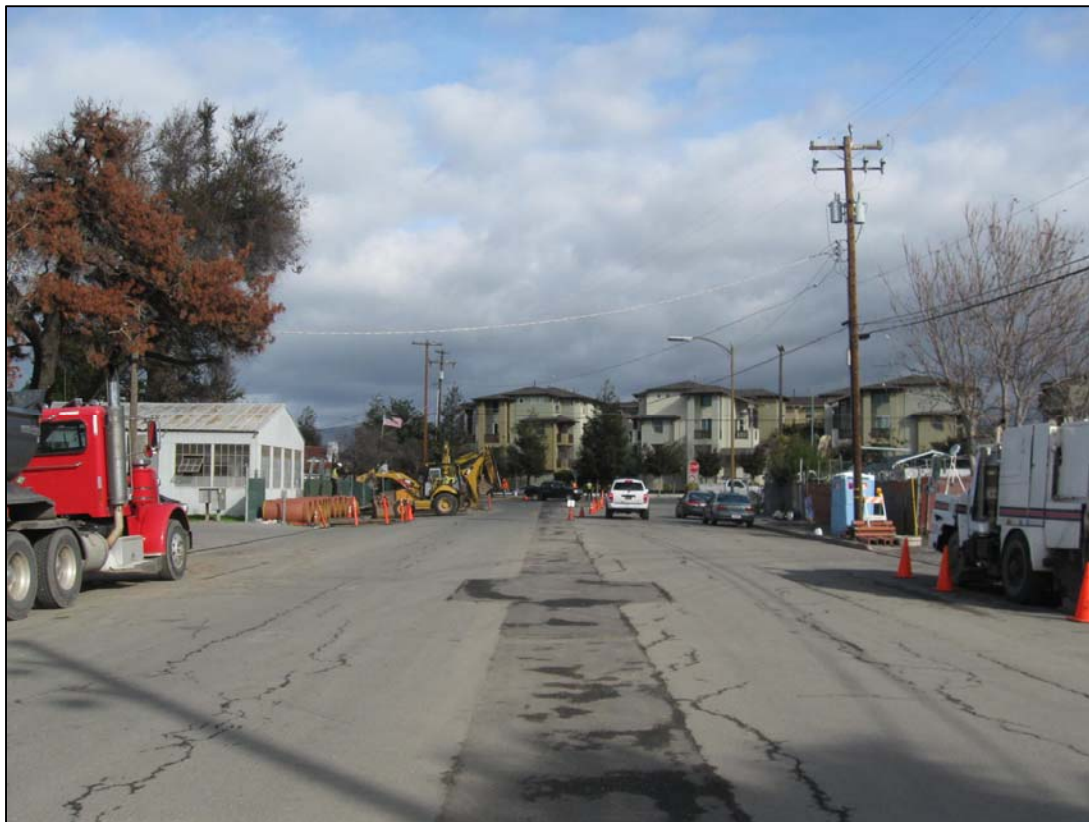
Photograph 10: Horning Street in front of the project site, facing east
