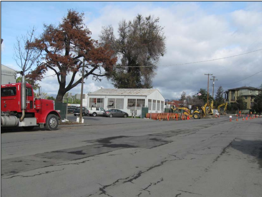
Photograph 1: The project frontage at 645 Horning Street, facing northeast
