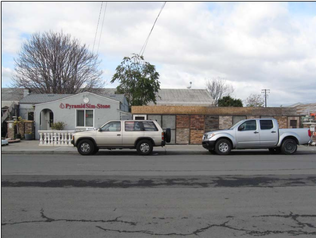
Photograph 5: Adjacent property to the west, facing north
