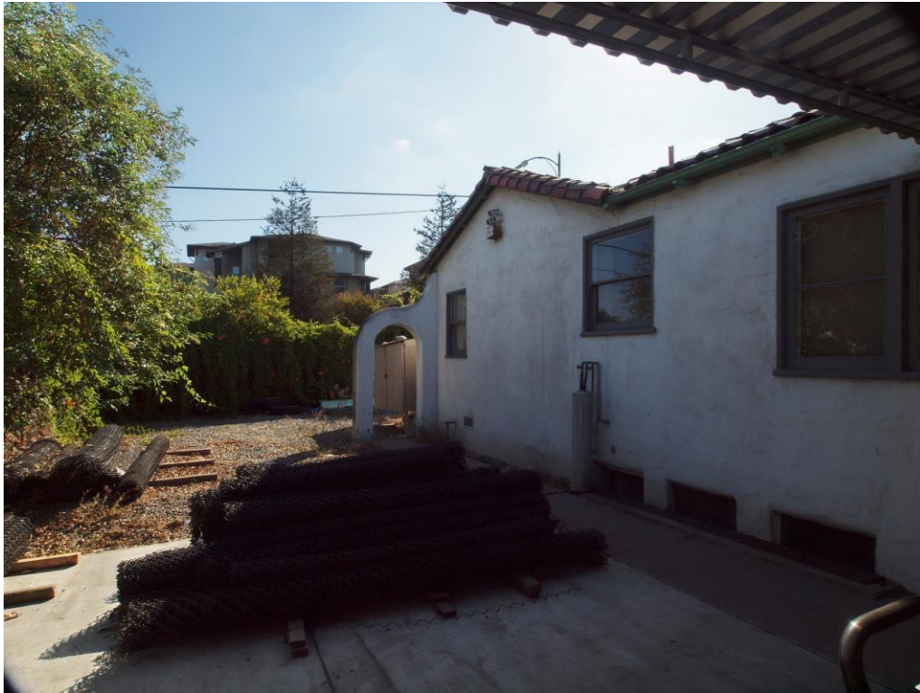
North elevation of house, viewed facing northeast.
