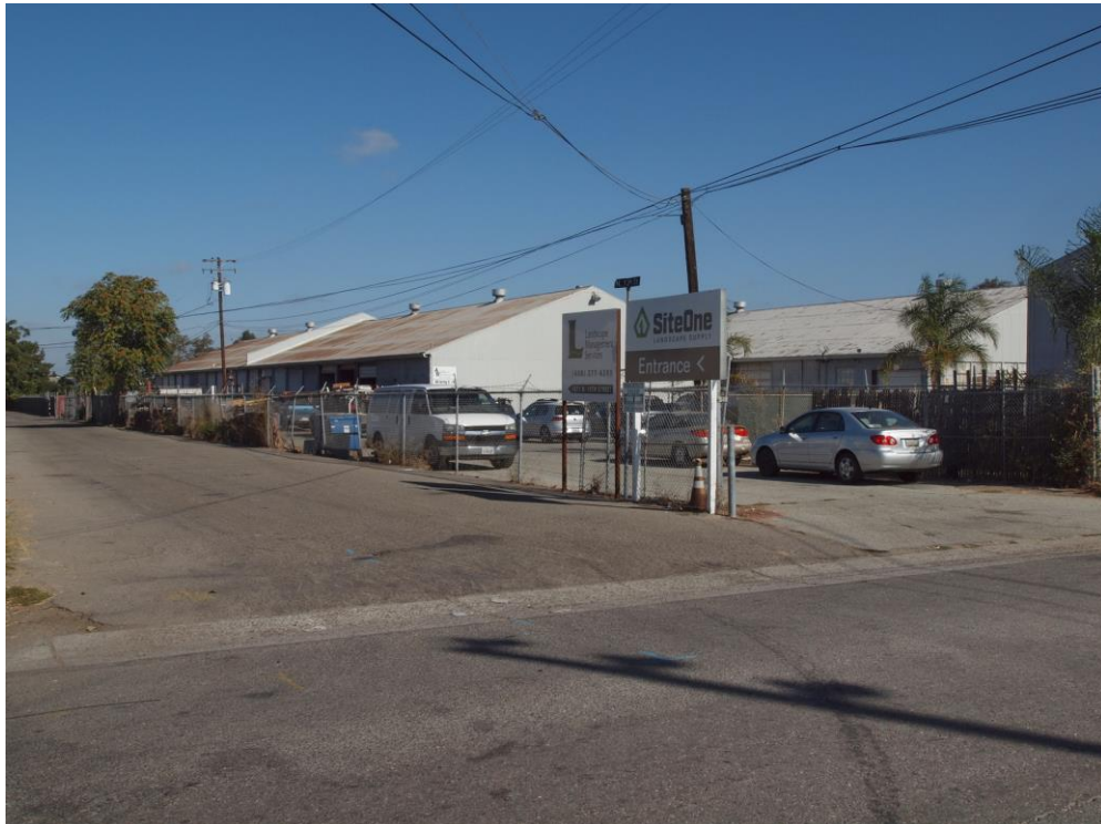
Truck storage structure (addition) viewed facing north.
