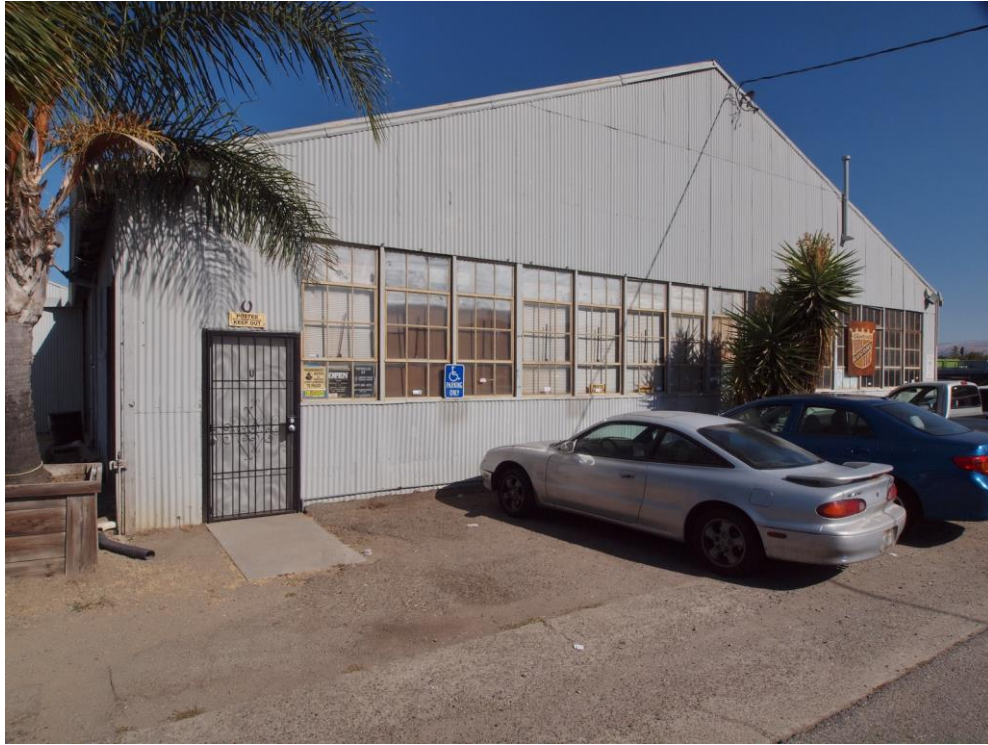
Front elevation of truck storage and repair structure, viewed facing north.
