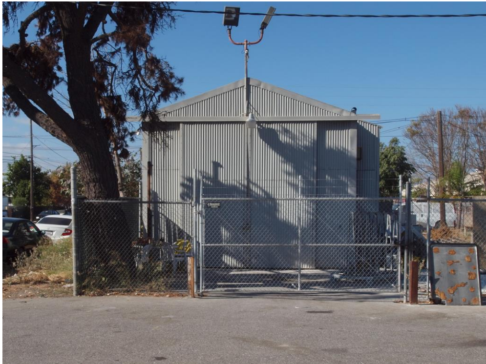
Second painting structure, viewed facing southwest.
