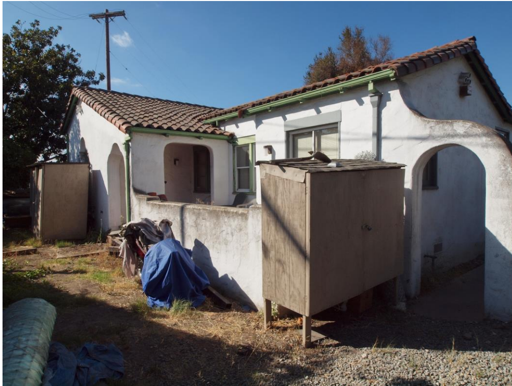
Front of house at 6435 Horning St., viewed facing southwest.
