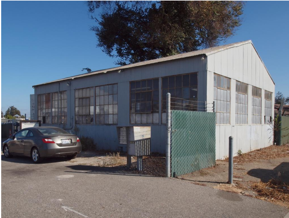
Original painting structure, viewed facing northeast.
