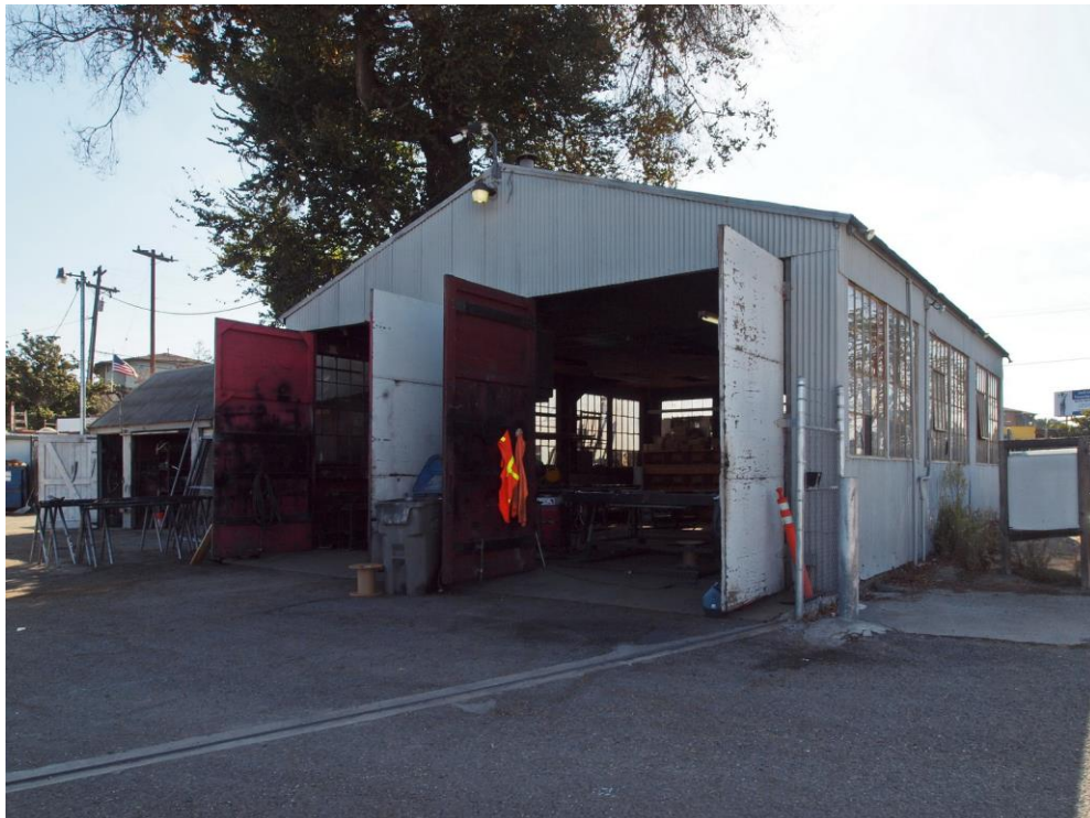
Original painting structure, viewed facing southeast.
