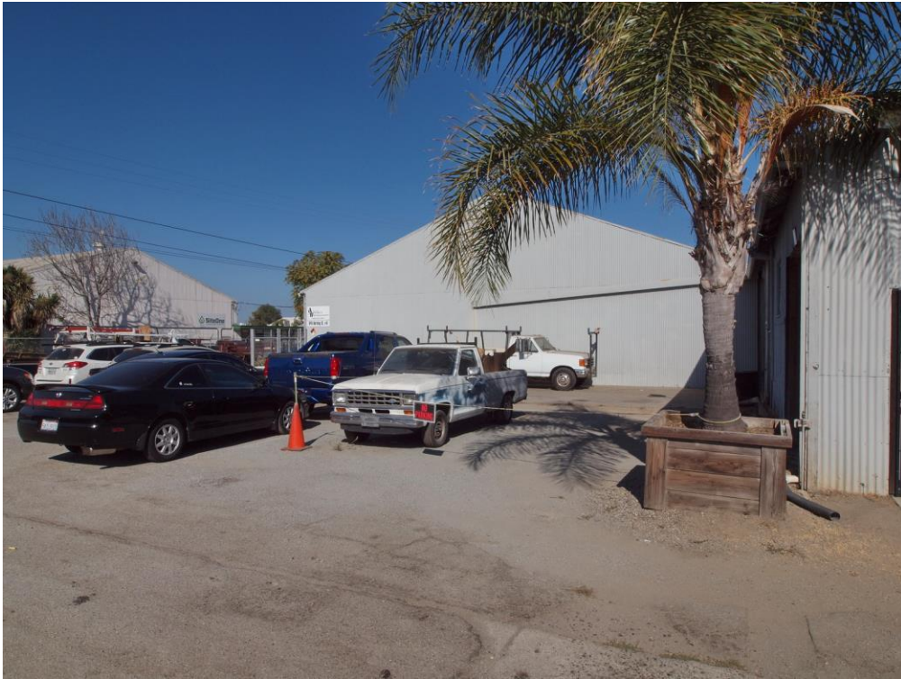
Truck storage structure (addition), viewed facing northwest.
