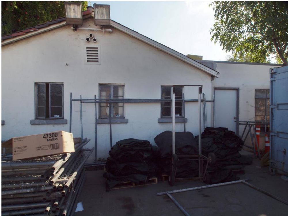
Rear elevation of office, viewed facing east.
