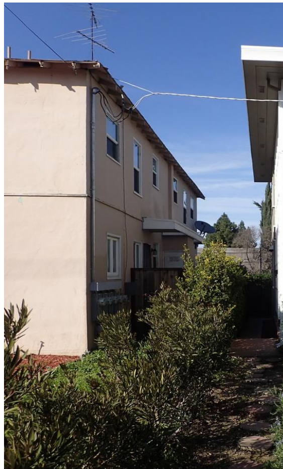
East side elevation at property line, viewed facing northwest.
