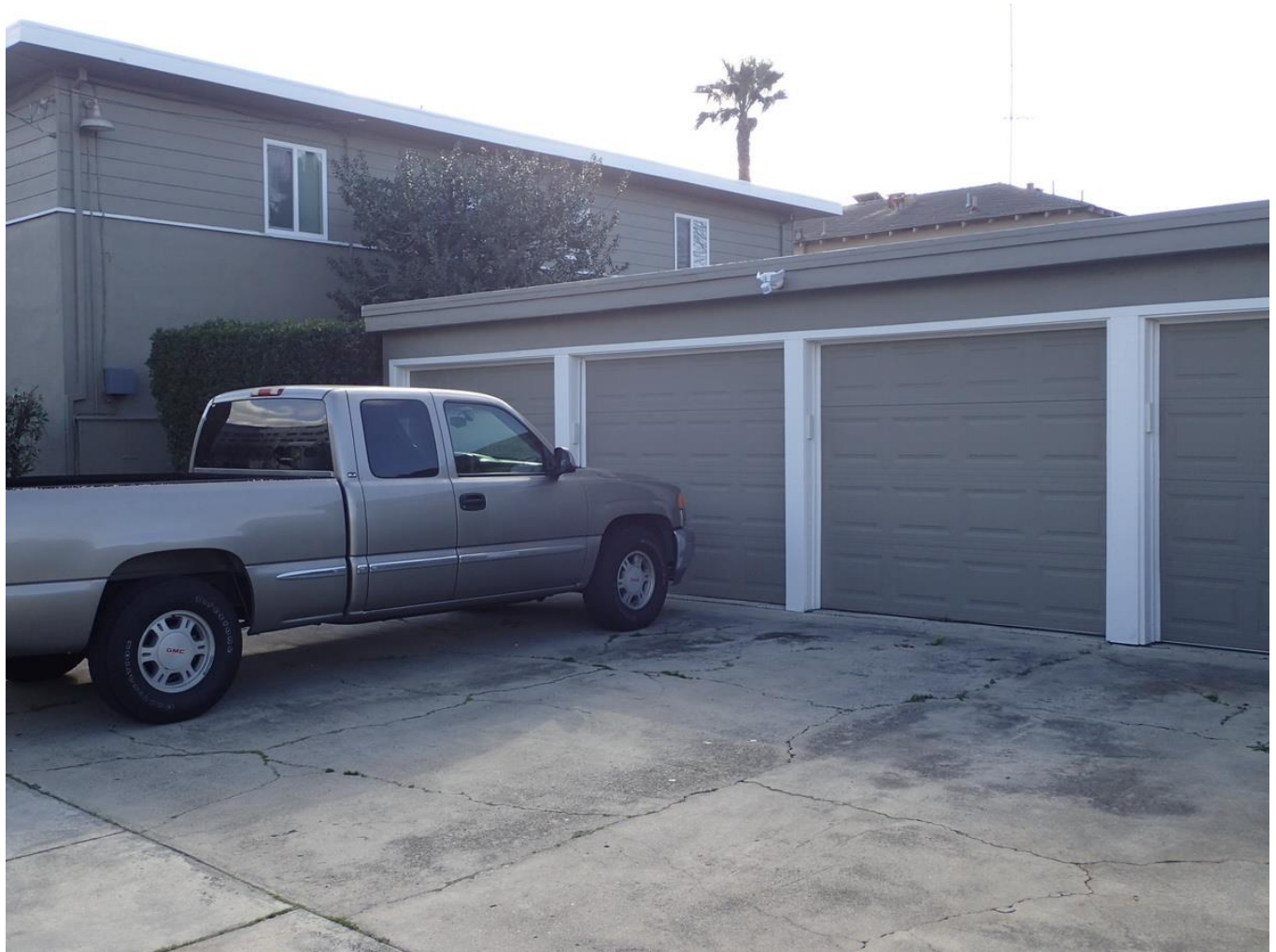
Garage structure at Central Way, viewed facing southwest.
