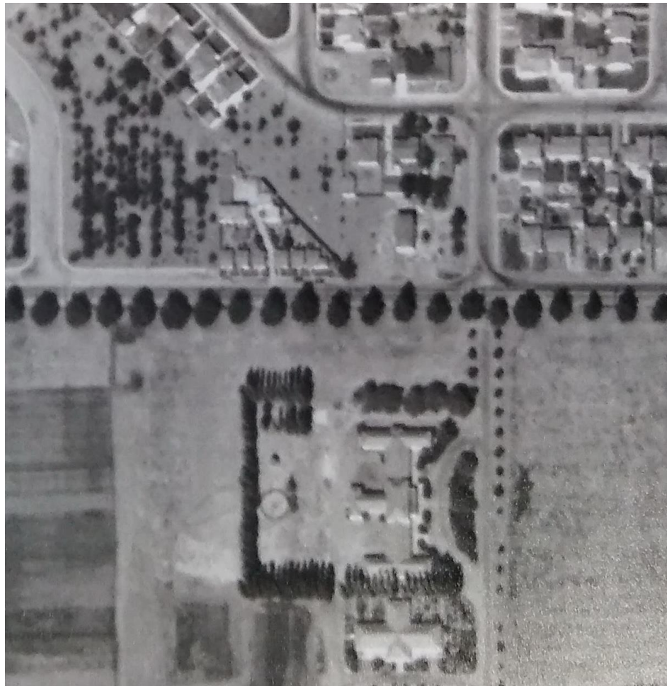
1948 USGS with the apartment building appearing to be under construction.
