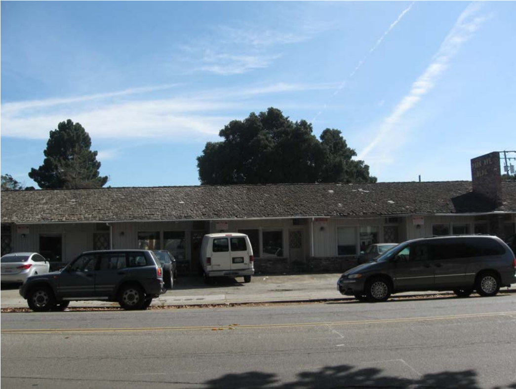
Photo 1: View of unoccupied office building on-site from Park Avenue, facing south
