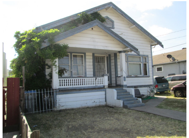
12. View of the subject property building at 246 Grand Avenue from the northwest
