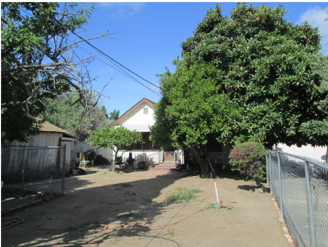
7. View of the subject property building at 245 Race Street from the east
