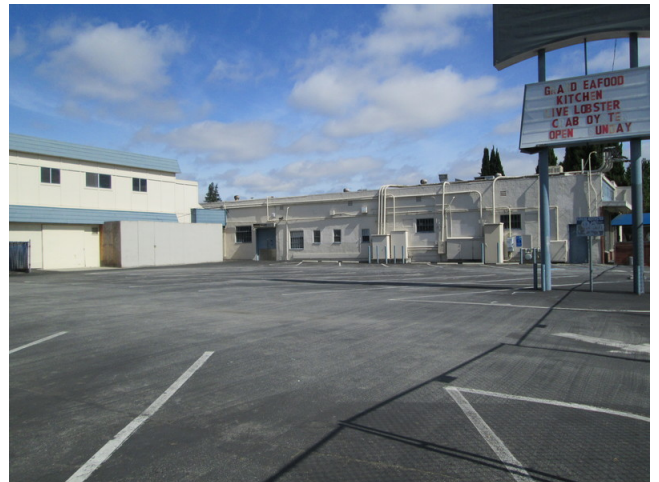
8. View of the subject property building at 253 Race Street/230 Grand Avenue from the southeast
