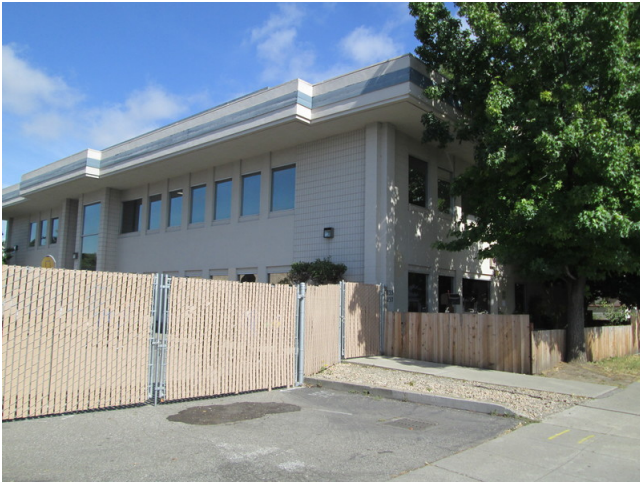
1. View of the subject property building at 237 Race Street from the southeast
