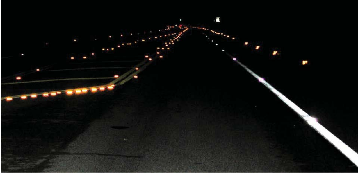
Figure 27. Embedded roadway lighting. These LED lights installed in the pavement are not visible to sea turtles nesting on the adjacent beach and are well received by motorists and pedestrians (Bertolotti and Salmon 2005). Photograph courtesy of Michael Salmon.
