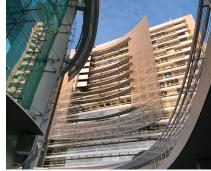
The "brise soleil" sunshading structure keeps the offices on the 18-story building's south side cool during the summer.
