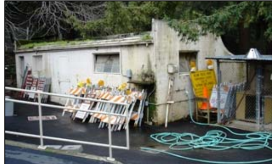
Figure 44: Restroom Building 7 (LSA)
