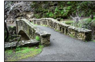
Figure 31: Pedestrian Bridge #2 (LSA)
