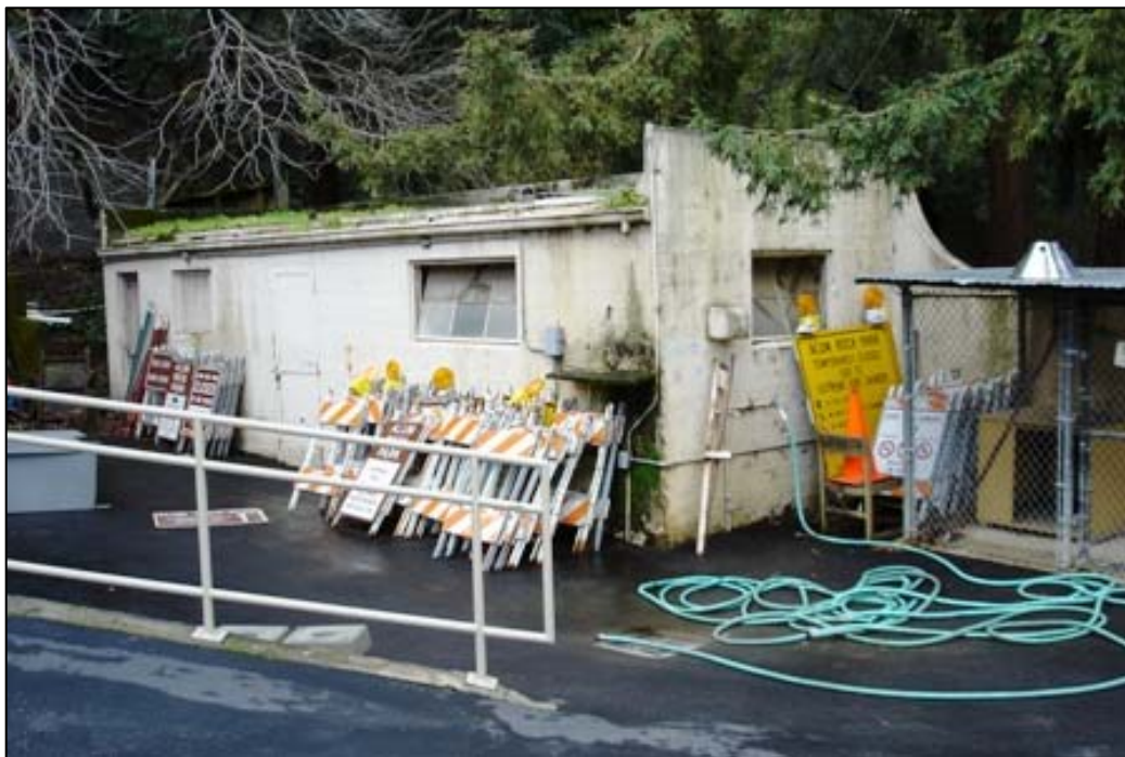
Natatorium Building. Restroom Building 7, northeast façades, view to the southwest.
