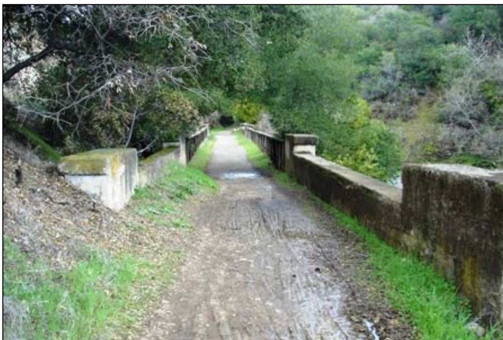
Pedestrian Bridge 5. Top of Trestle. View of old Southern Pacific railroad bed, view to the SW.
