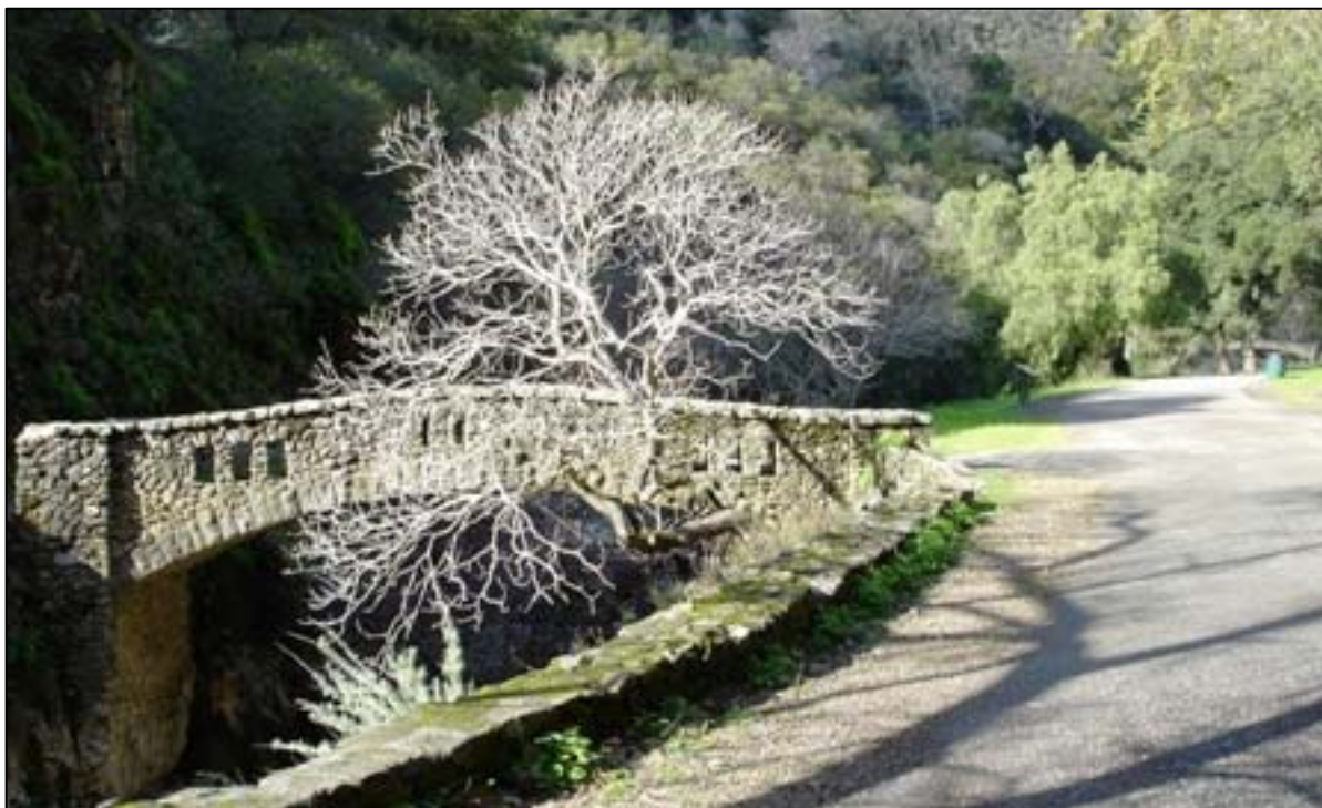
Pedestrian Bridge 2. View East. Pedestrian Bridge 1 visible in background.
