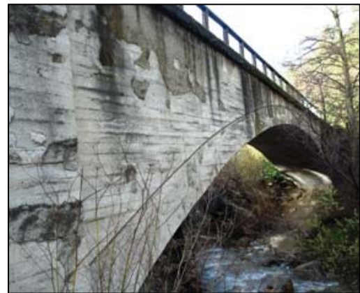
Figure 9: Pedestrian Bridge 5 (LSA)
