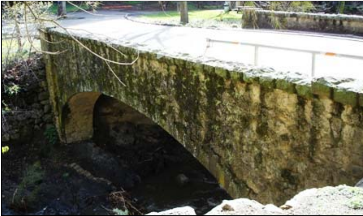
Alum Rock Bridge. View to the SW.
