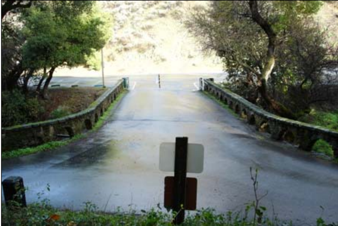
North View of bridge deck.
