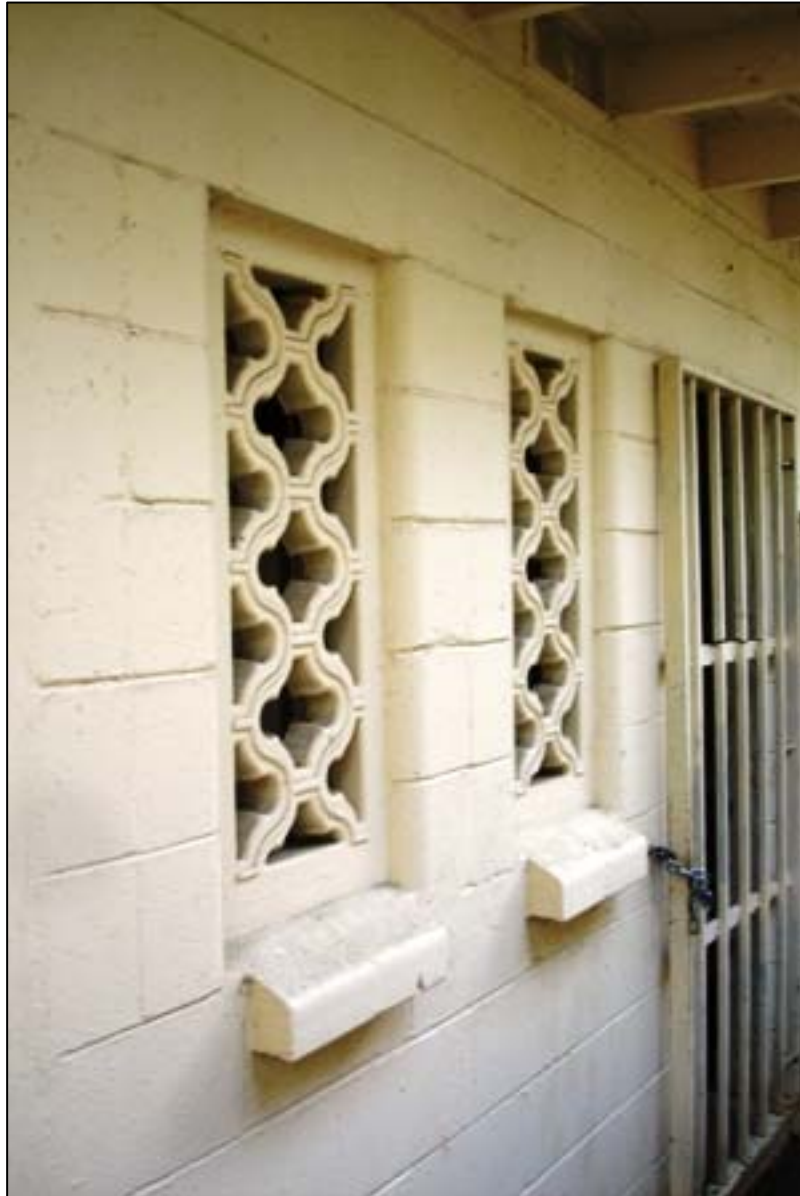
Restroom Building 1. Windows.
