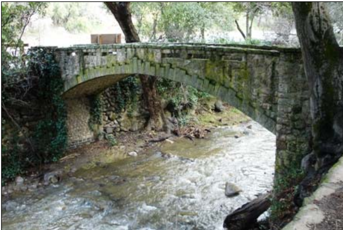
Pedestrian Bridge 3. View NE.
