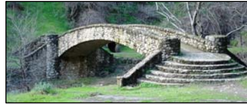
Figure 30: Pedestrian Bridge #1 (LSA)
