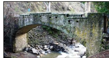
Figure 33: Pedestrian Bridge #4 (LSA)
