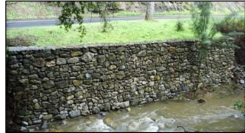
Figure 39: Masonry Retaining Wall (LSA)
