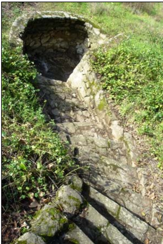
(left) open clam-shell Reservoir.
