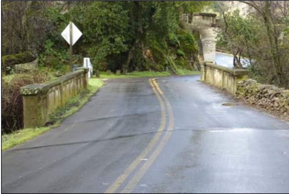
West facing view of bridge deck.
