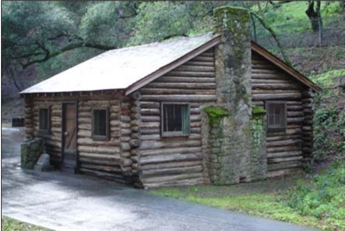
Log Cabin. Northwest façades. View to the southeast.
