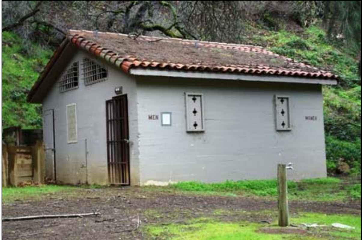
Restroom Building 3, northeast façades, view to the southwest.
