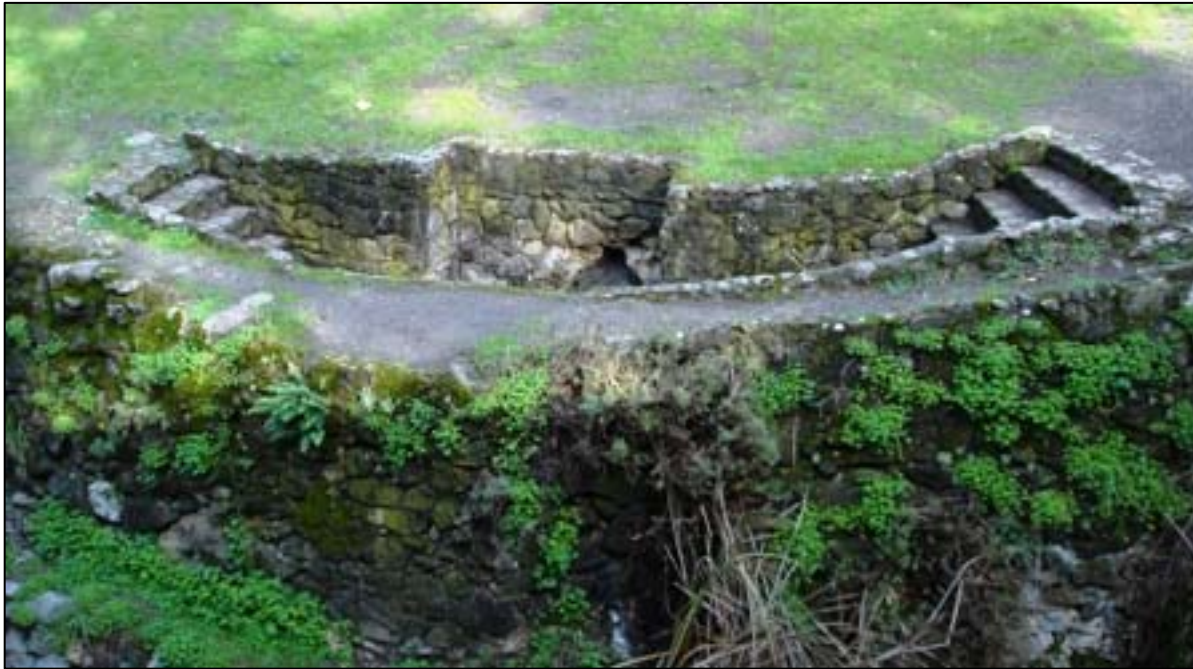
Clam-shell reservoir. View south.
