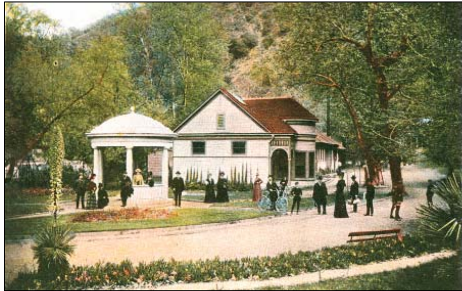
Figure 6: Historic Bathhouse and Gazebo (1900-1910).*
