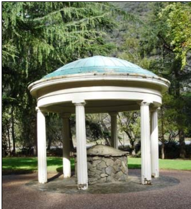
(left) Gazebo. View to the NE.
