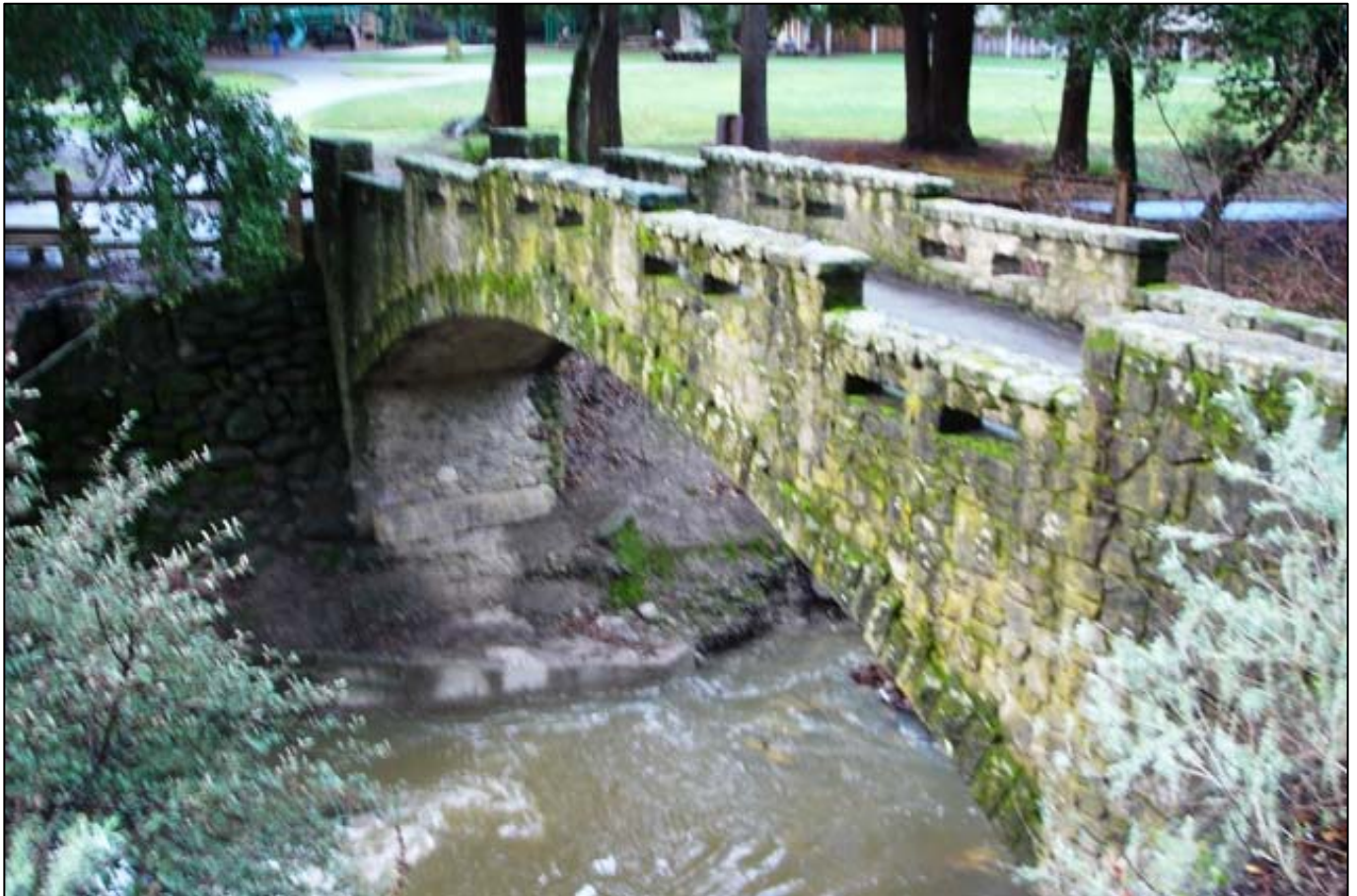
Pedestrian Bridge 4. View across Penitencia Creek. Natatorium site in background. View SW.
