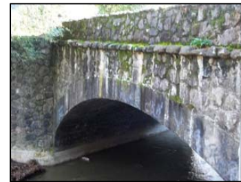
Figure 24: Automobile Bridge #1 (LSA)
