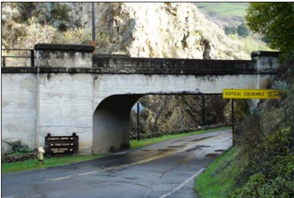
Pedestrian Bridge 5. Alum Rock Falls Road span. View NE.
