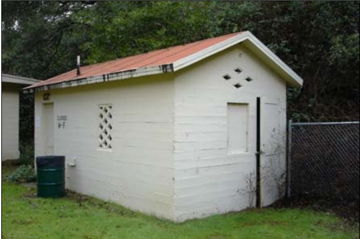
Restroom Building 2. Southwest façades, view to the northeast.
