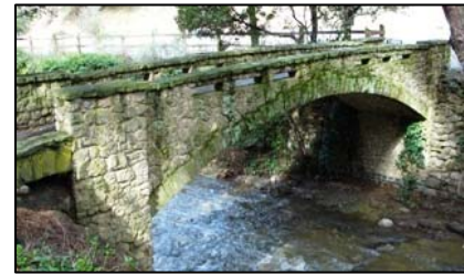
Figure 32: Pedestrian Bridge #3 (LSA)
