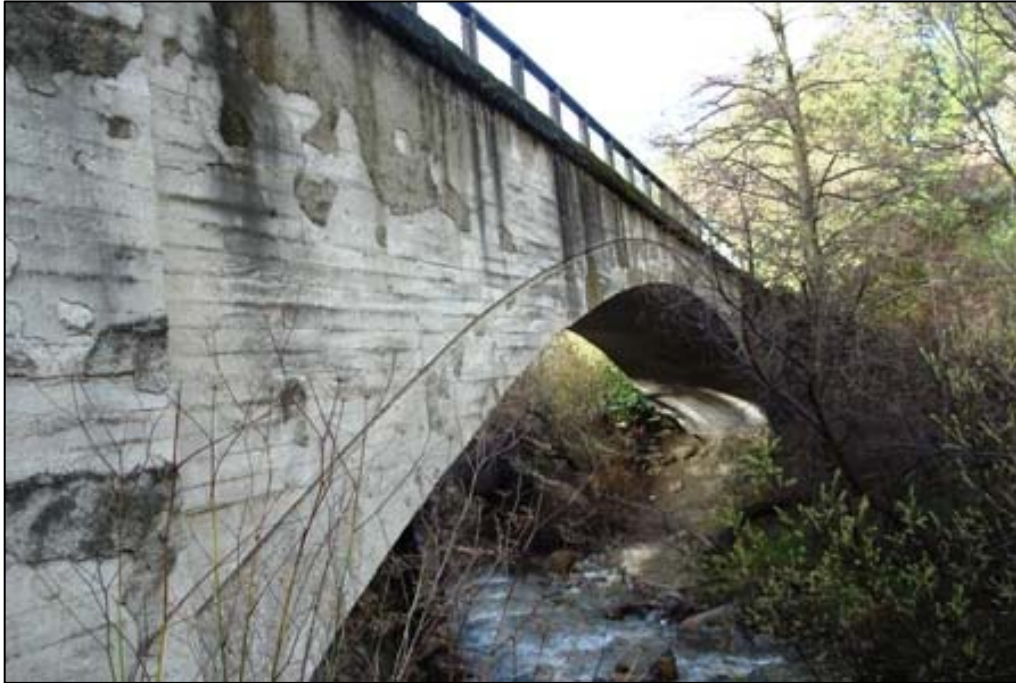
Pedestrian Bridge 5. Penitencia Creek Span. View to the West.
