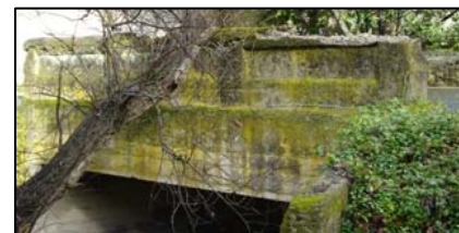
Figure 25 Automobile Bridge #2 (LSA)
