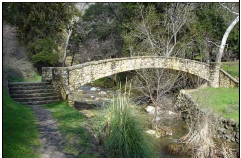
(below) Pedestrian Bridge 1: view east.
