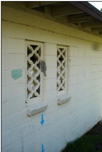
Restroom Building 5. North façade, window detail.
