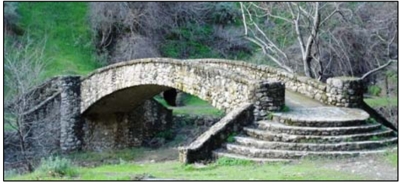
Figure 11: Pedestrian Bridge 1 (LSA)
