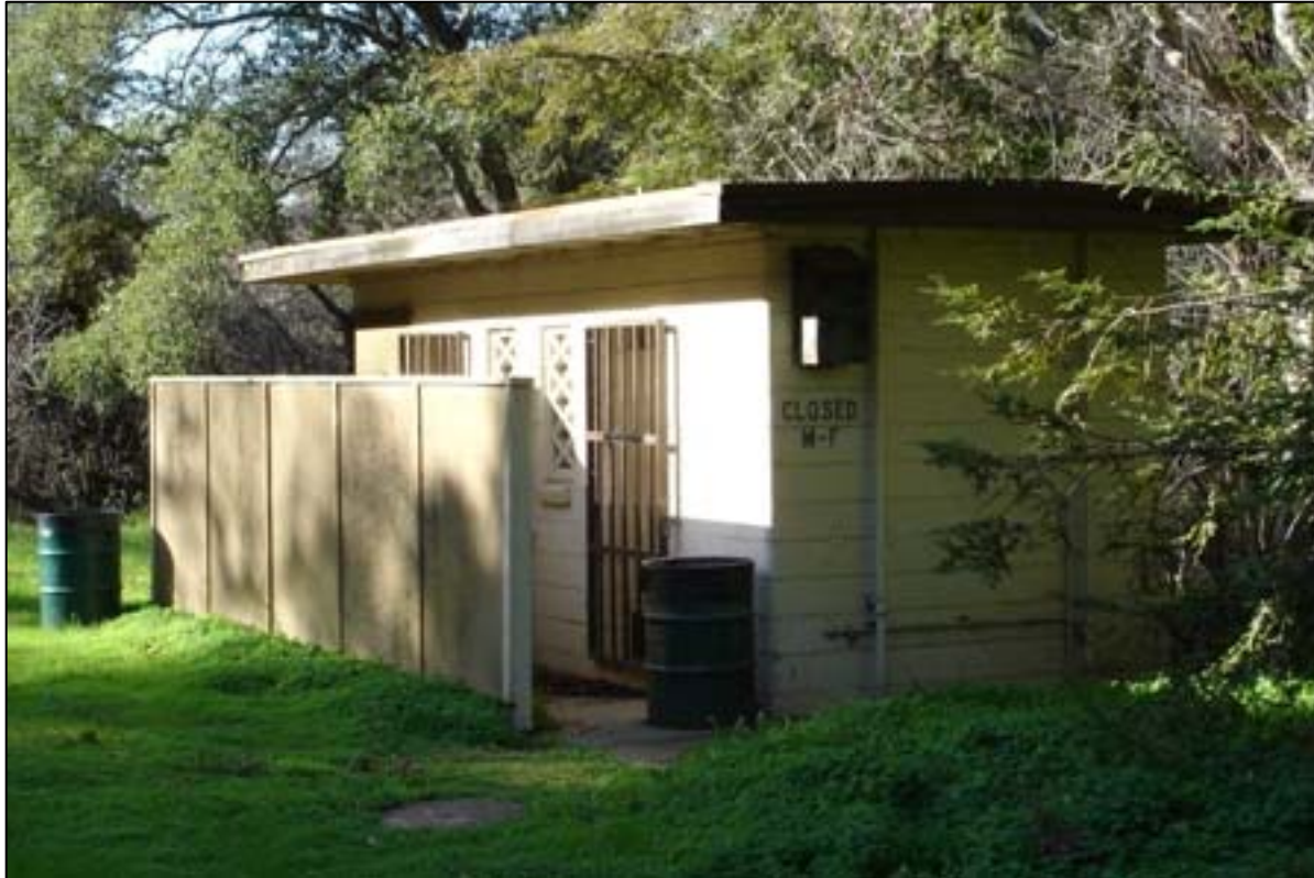
Restroom Building 6. Southeast façades, view to the northwest.
