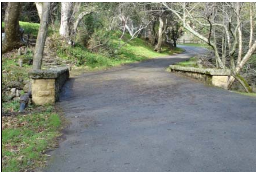
Automobile Bridge 6. View of bridge deck, facing east.
