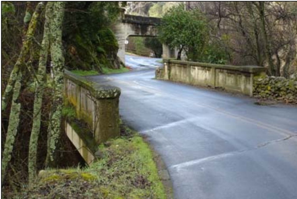
Northwest facing view of bridge deck.
