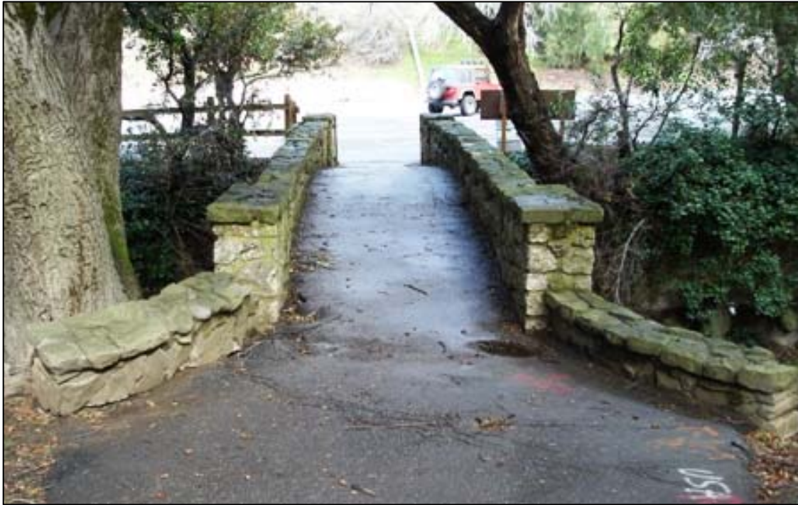
Pedestrian Bridge 3 bridge deck. View North.
