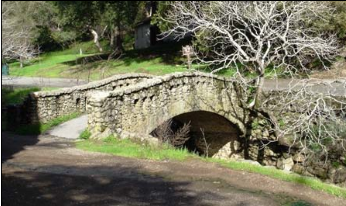
Pedestrian Bridge 2. View SE.
