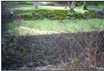
Figure 38: Masonry Retaining Wall (LSA)
