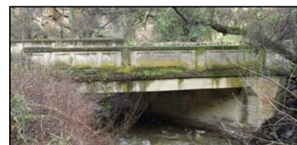
Figure 26: Automobile Bridge #3 (LSA)
