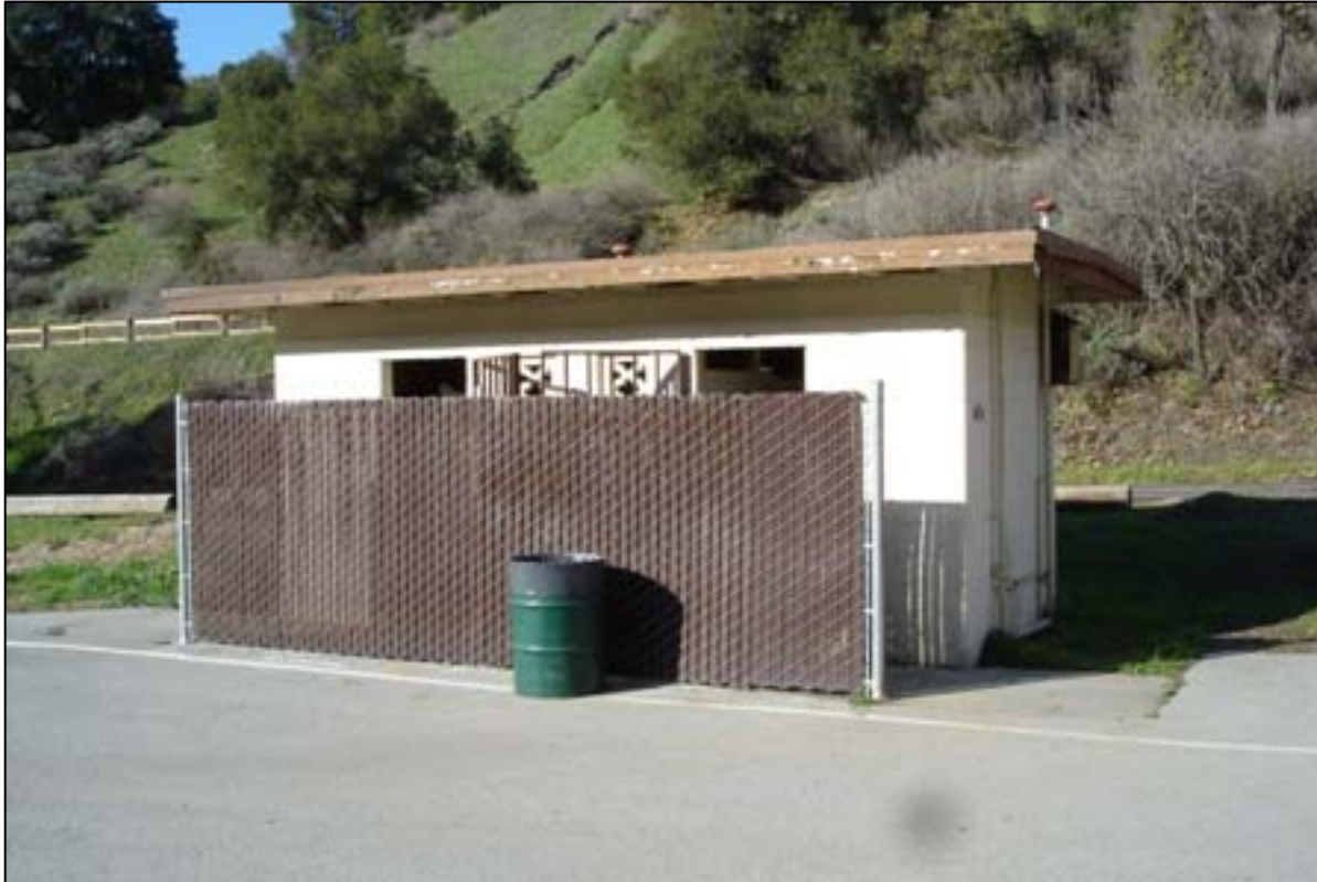
Restroom Building 5. Southeast façades, view to the northwest.
