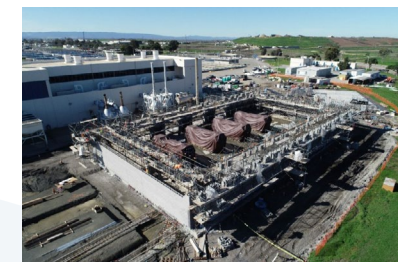
New Cogeneration Facility in construction
