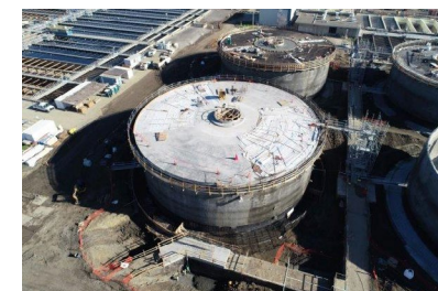
Thermophilic Digesters in construction
