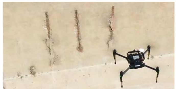
Figure 4: Drone inspection of Aeration Tanks
