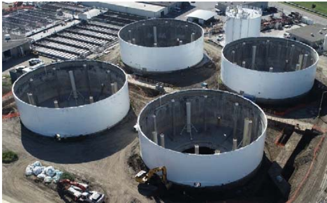
Figure 2: Photograph of digesters taken by the drone
