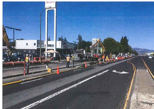
Stevens Creek Blvd Pipe Installation
