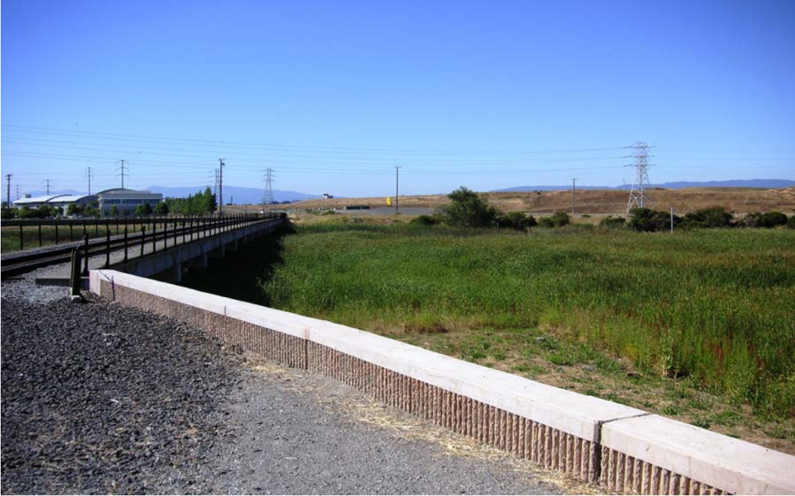
Looking south from approximate pedestrian structure northerly touchdown point, UPRR structure to east.
