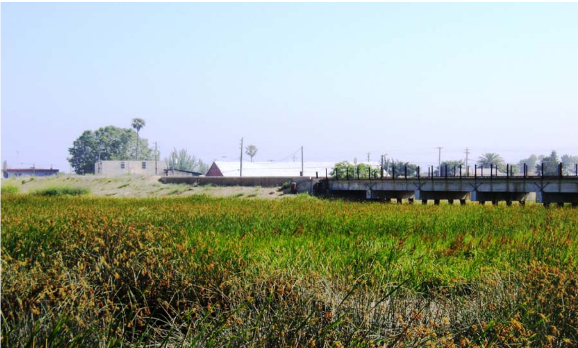
Looking north at approximate pedestrian structure northerly touchdown point, UPRR to east.
