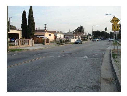
As shown in the picture above, the markings on the road bumps are faded. Therefore, although the road bump warning sign is visible, and at night the reflective markers at the base of the road bumps are visible, the road bump markings are not clearly visible. We visited another location with road bumps. The following picture shows a road bump that was installed in April 2006.
