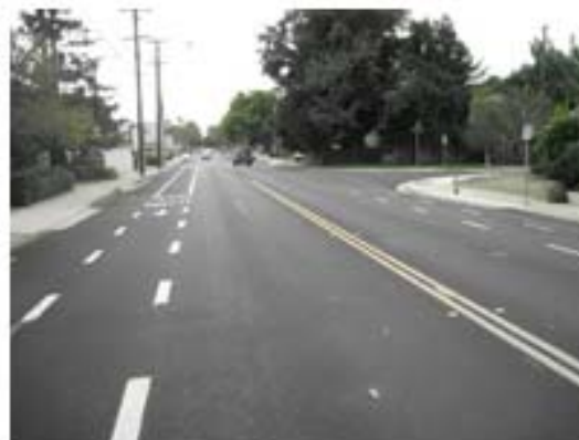
Willow Street after street resurfacing (Tier 1)
