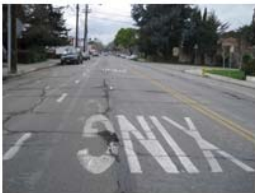
Willow Street before street resurfacing (Tier 1)
