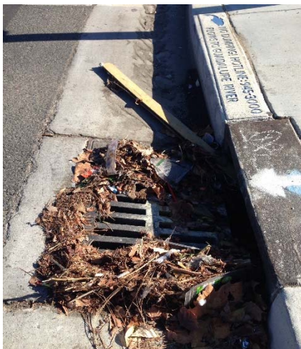
↑ Litter and debris apparently conveyed to a storm drain from the previous day's rain. November 3, 2015.
