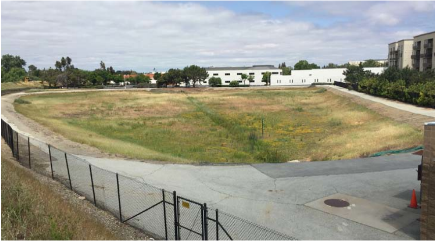
River Oaks Pump Station
