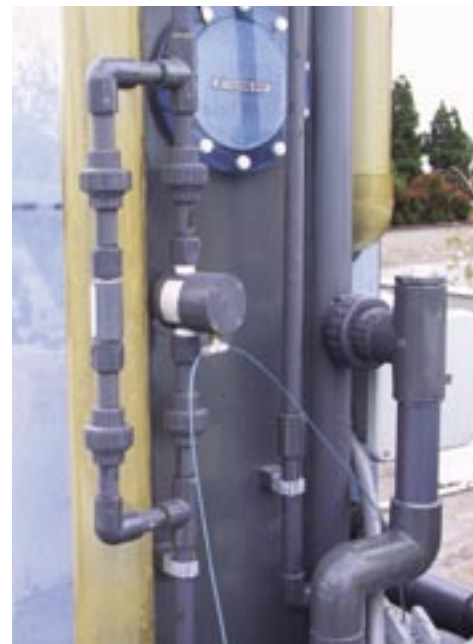
The fume scrubbers — which operate at all times — contributed close to 80% of Reaction Technology's total water use.
