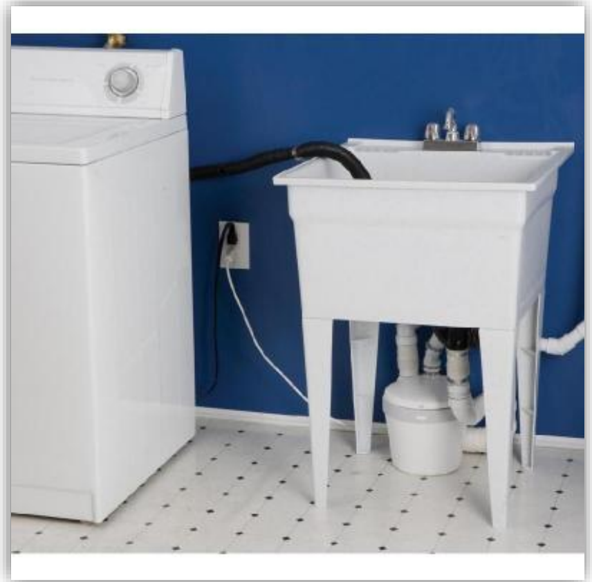
A hose directing wastewater to a utility sink, which drains into the sewer system.
