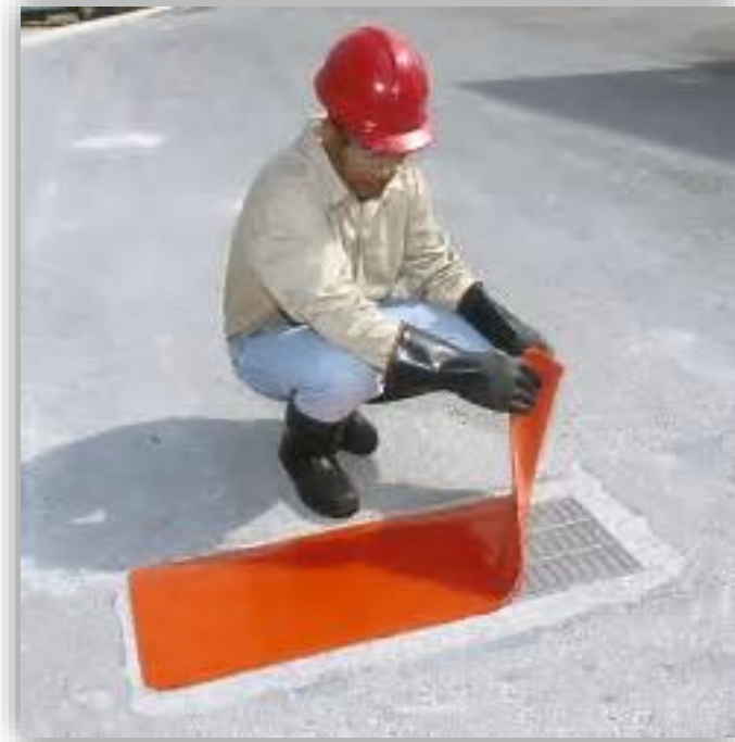
A storm drain covered with a mat.
