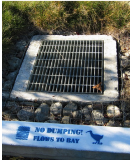
Only rain should flow down the storm drain. Storm drains flow directly to creeks and the Bay.
