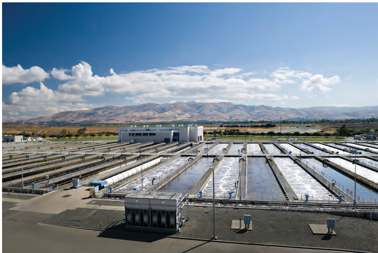
Eastward view of the secondary treatment tanks that use bacteria to clean wastewater.
