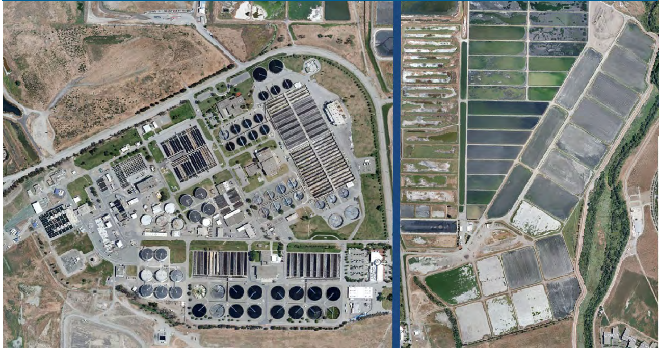
Existing Plant and residual solids management areas
