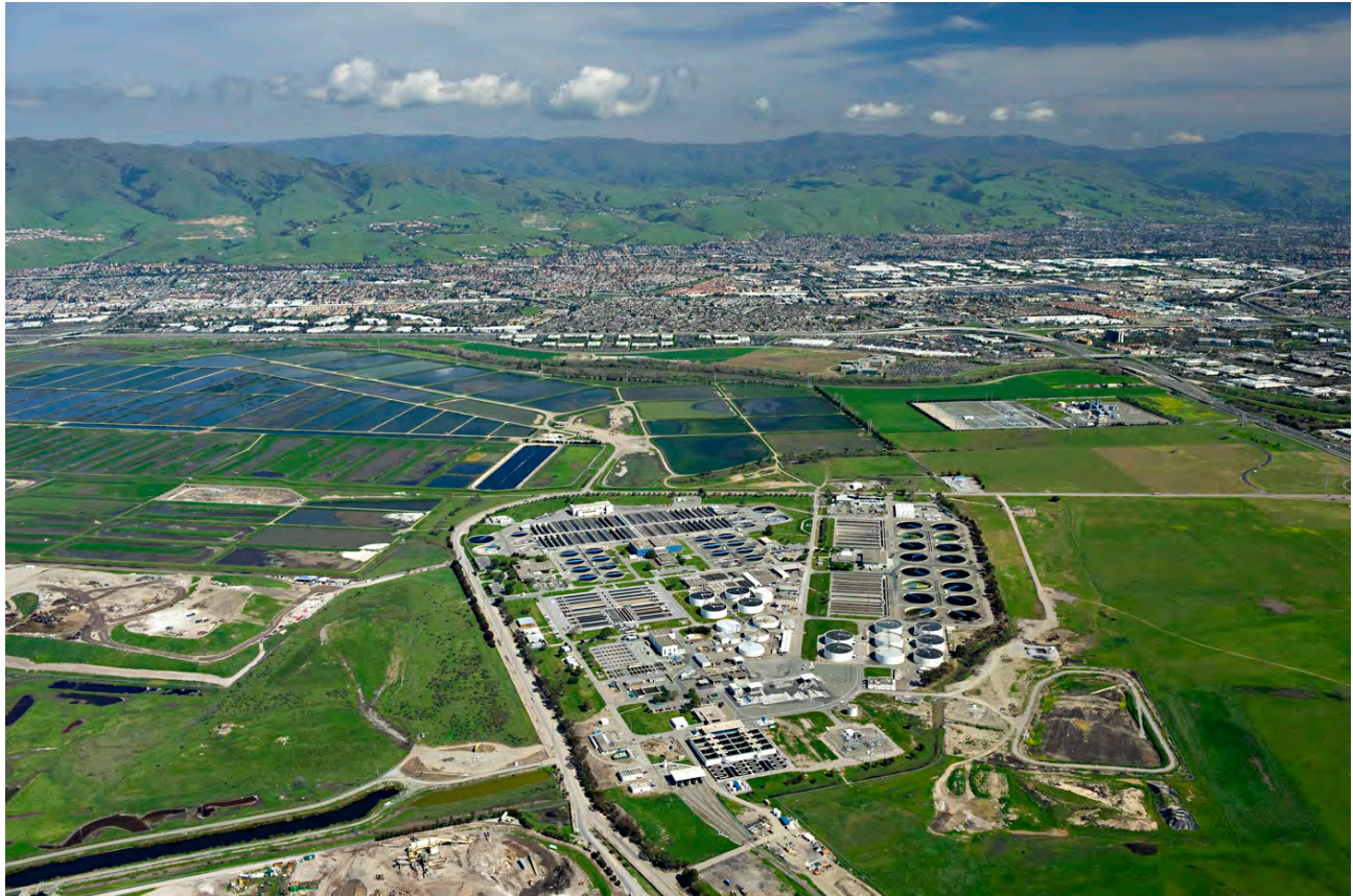
Aerial view of Plant site looking eastward.
