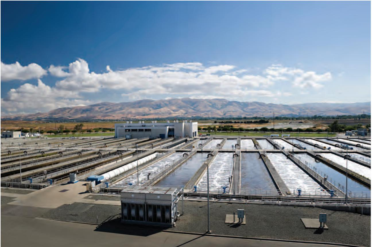
*Eastward view of the secondary treatment tanks, which use bacteria to clean wastewater.*
