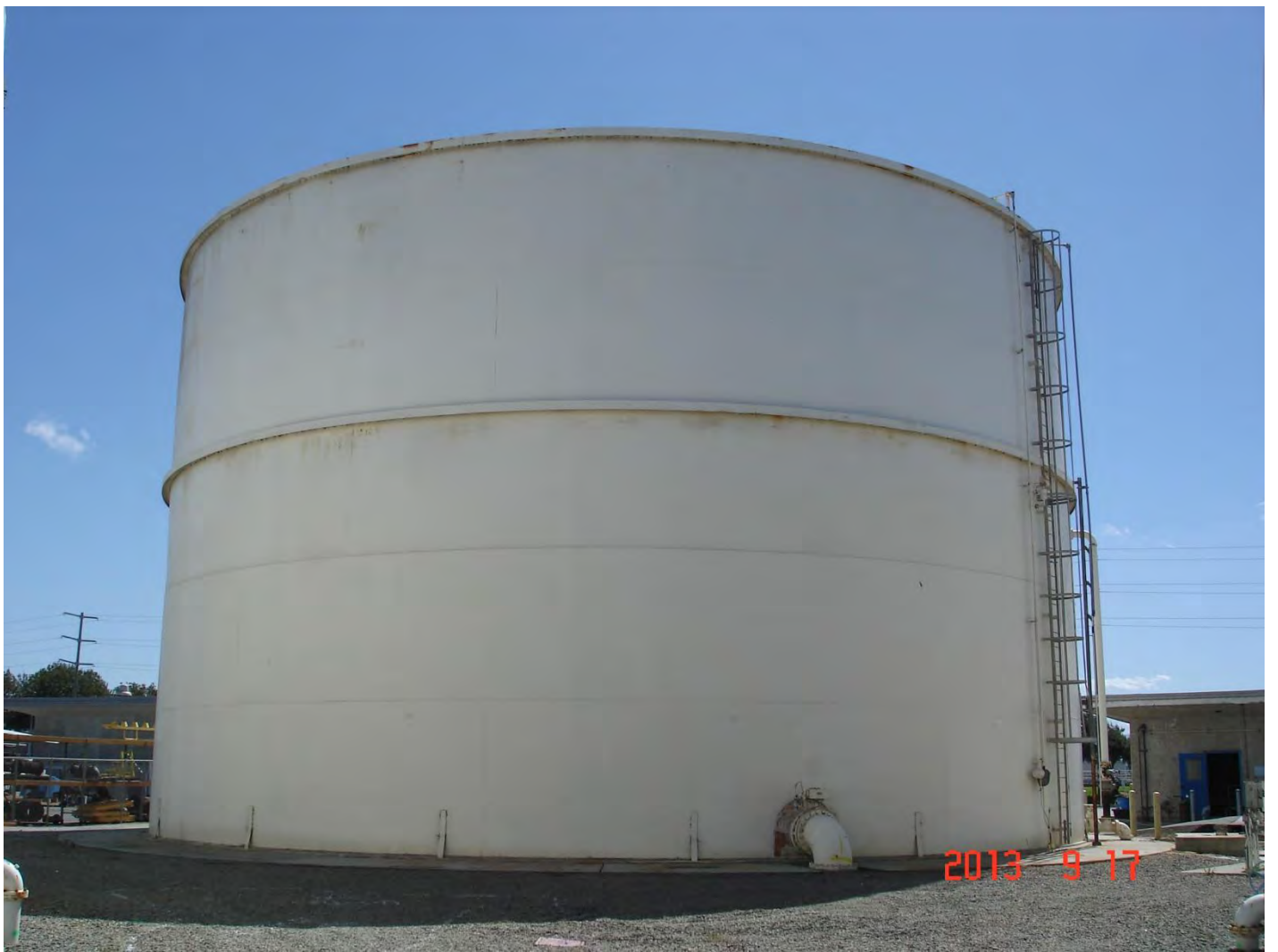
Figure 3: Existing Gas Storage Tank
