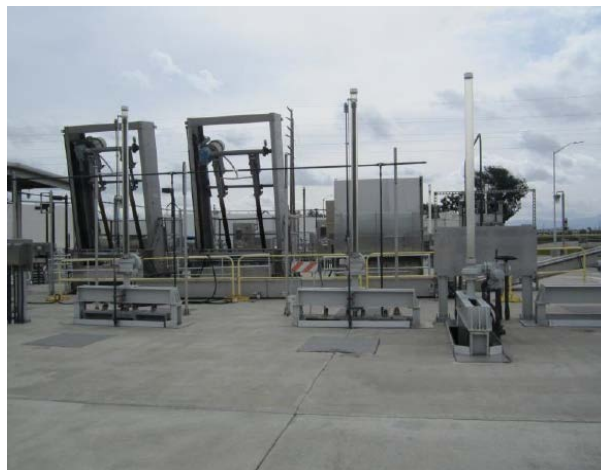
Figure 3 – Existing Headworks 2 Facility
