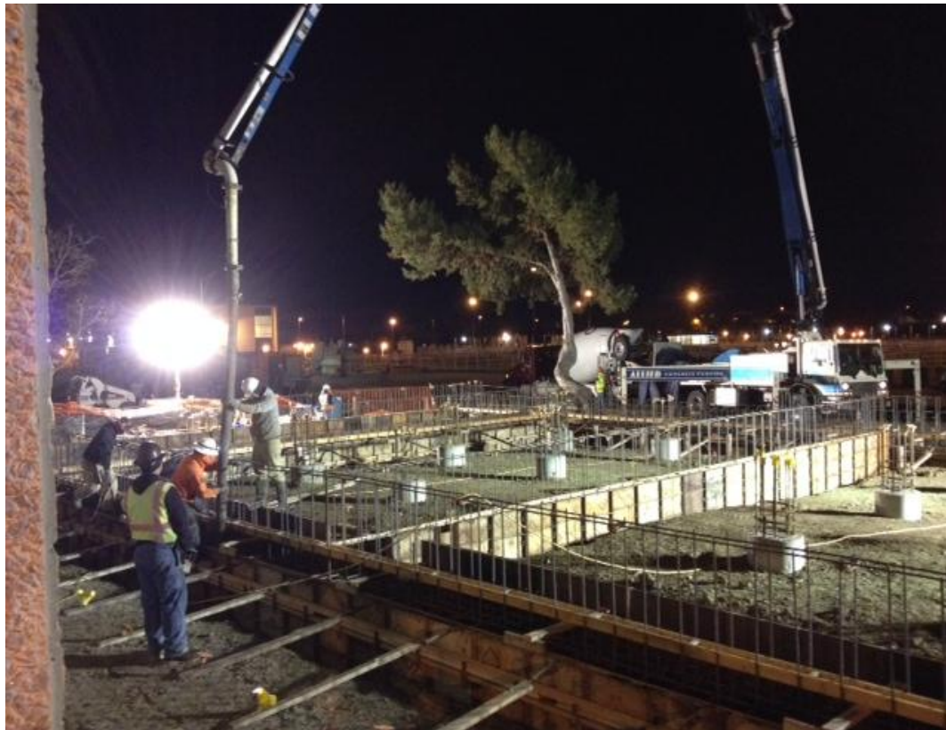
Figure 3: Grade Beams/Footings Concrete Pouring in Progress
