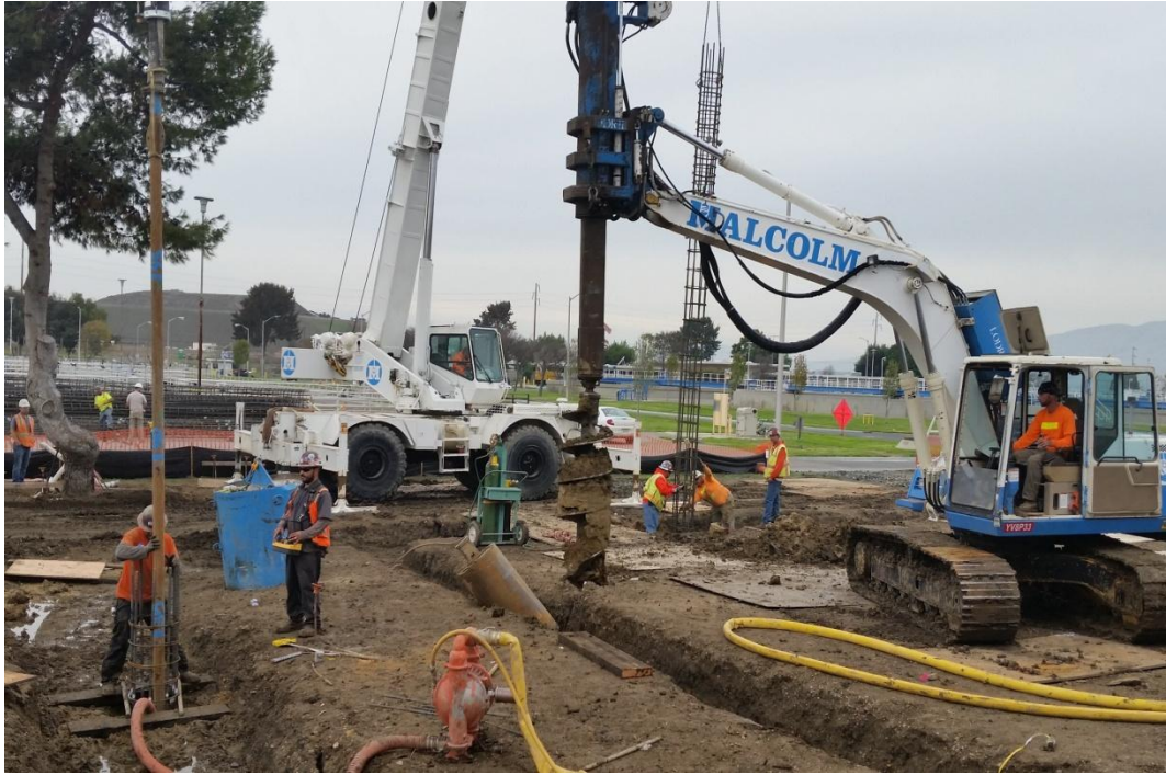
Figure 2: Pier Construction in Progress
