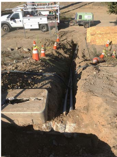
Figure 3: New conduits at Hwy 237 and Zanker Rd
