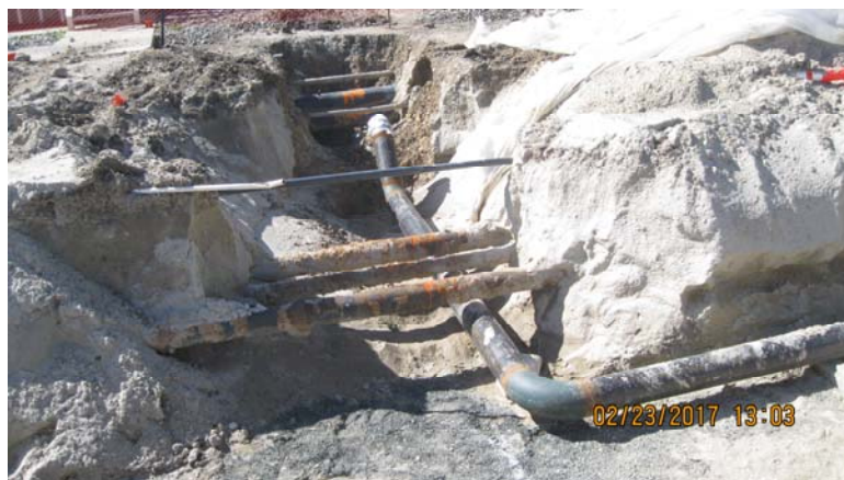
Figure 2: Underground Utility Routing Challenges
