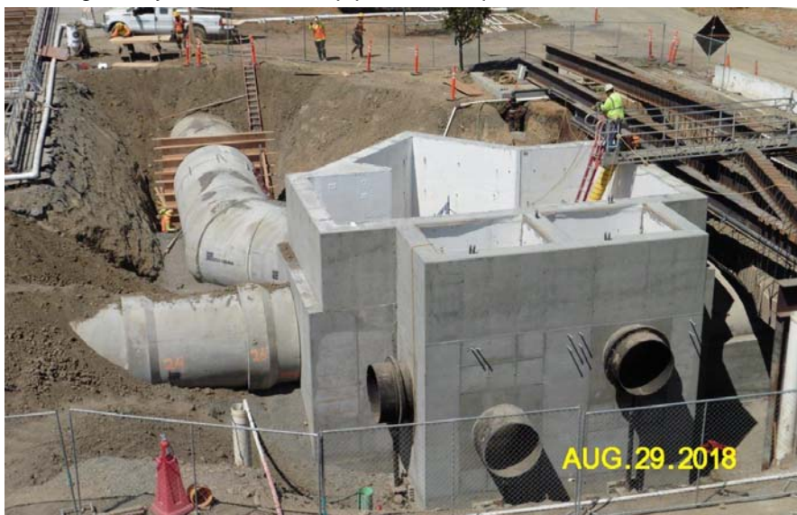
Figure 2: New wye structure
