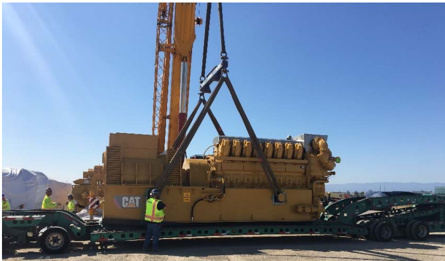
Figure 1: Unloading Caterpillar CG260-16 engines at the RWF
