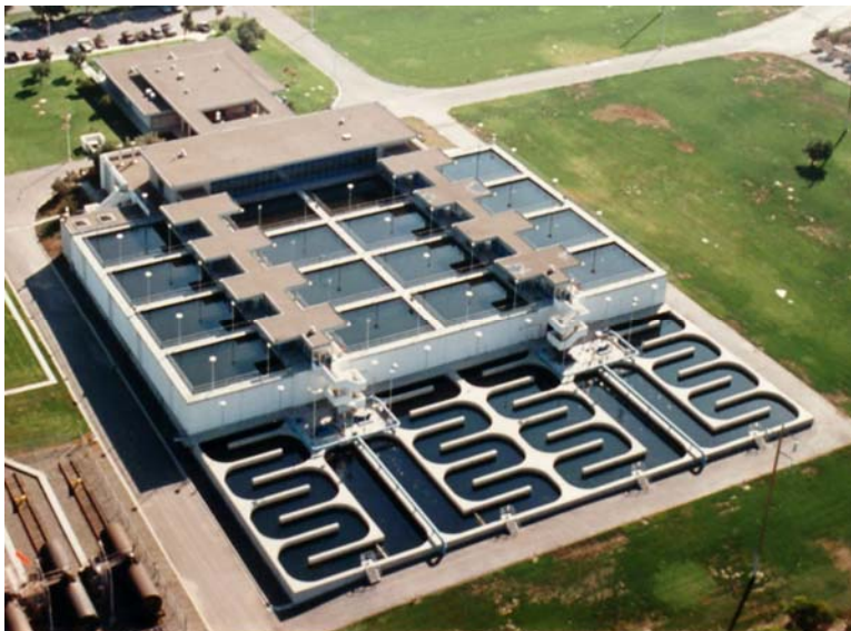
Figure 3: Filter Building, Filter Beds, and Serpentine Tanks
