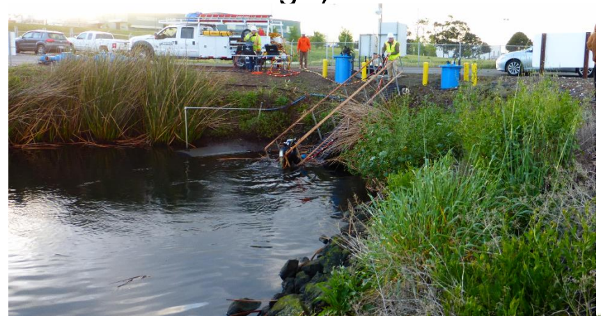
A diver inspected flow meters inside outfall pipes in 2018.
