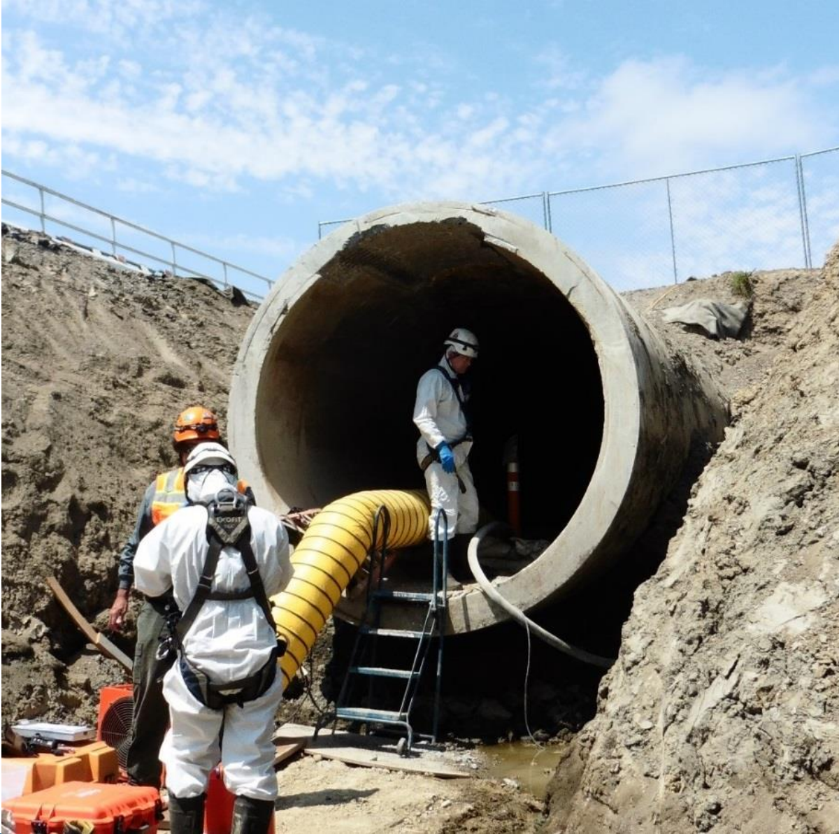
96-inch and 87-inch Settled Sewage (SES) Pipe Rehabilitation
