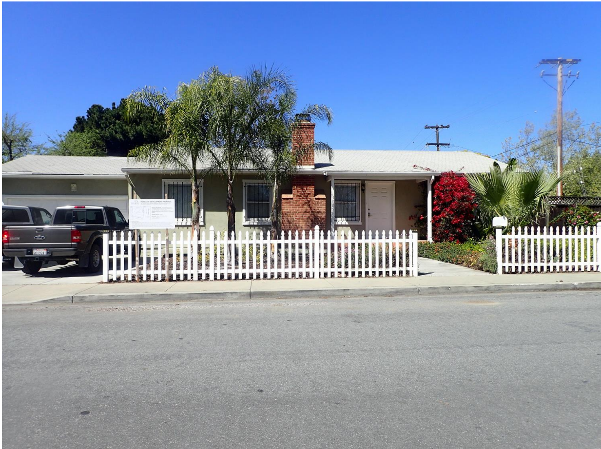
View from Hemlock Avenue facing north.
