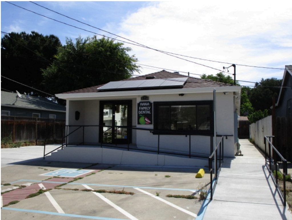
28. Hana Family Dental (374 South Redwood Avenue) adjacent to the west
