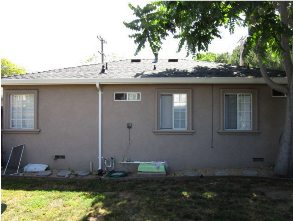
3. Western side of the 375 South Baywood Avenue residence
