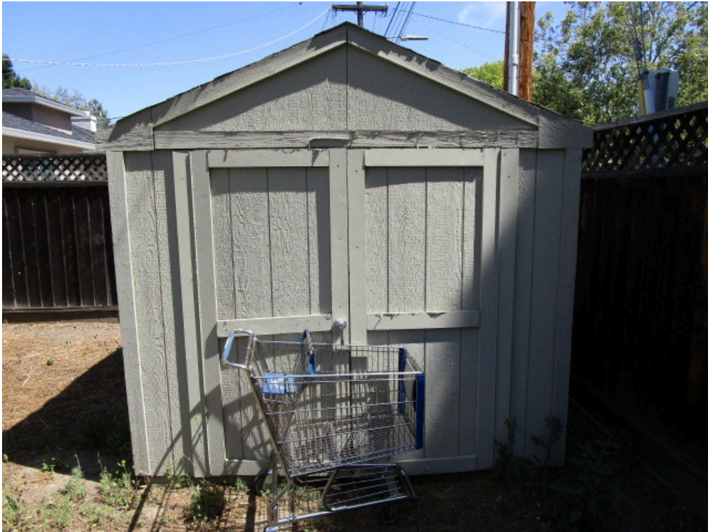
13. 383 South Baywood Avenue residence - shed
