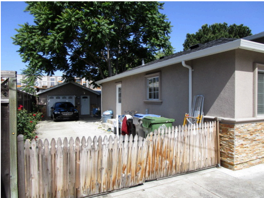
2. Driveway and southern side of the 375 South Baywood Avenue residence
