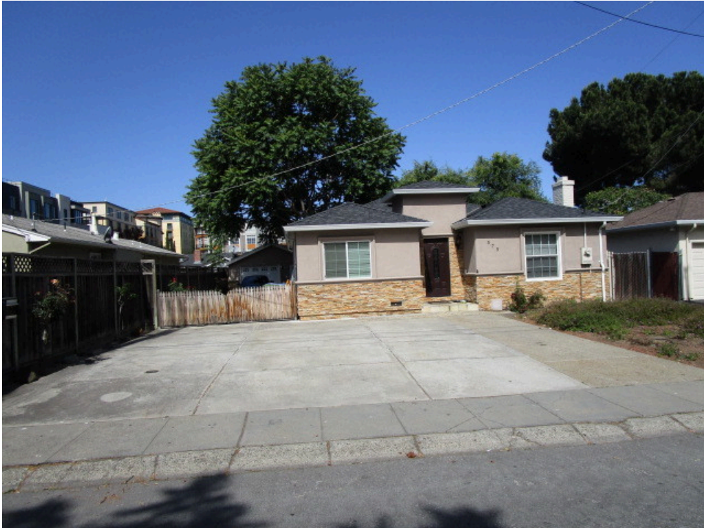
1. Eastern side of the 375 South Baywood Avenue residence
