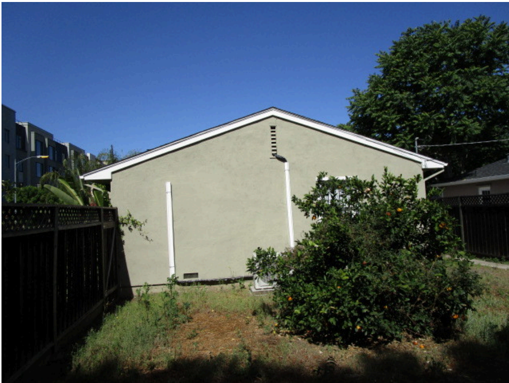
10. Eastern side of the 383 South Baywood Avenue residence
