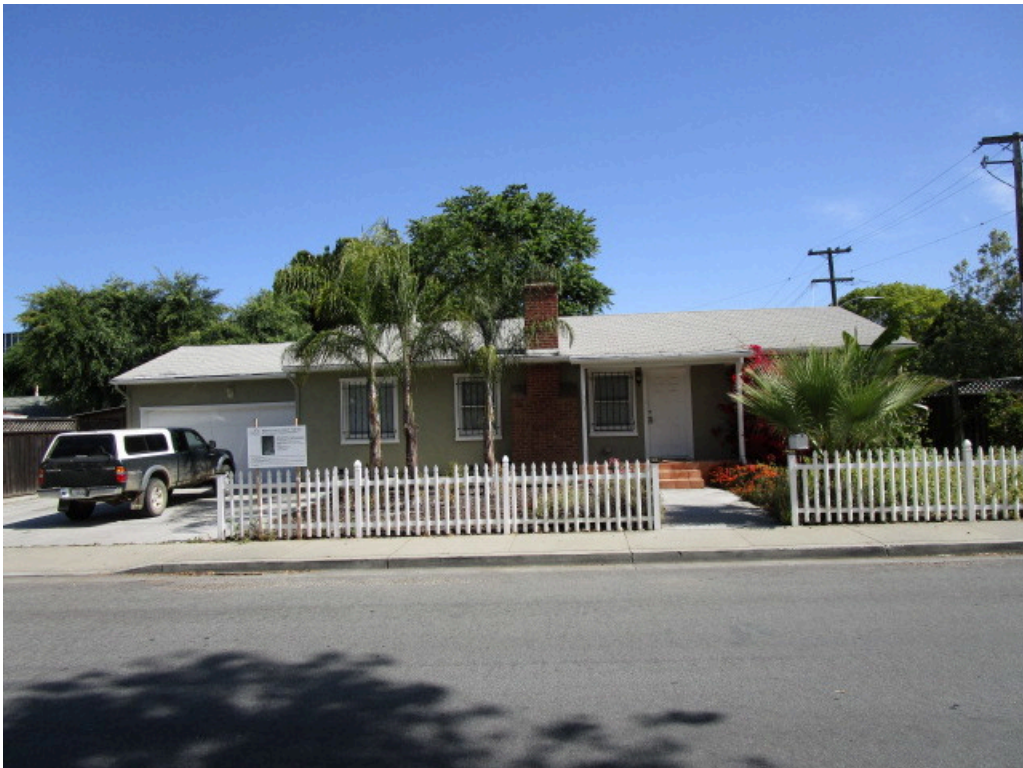
8. Southern side of the 383 South Baywood Avenue residence
