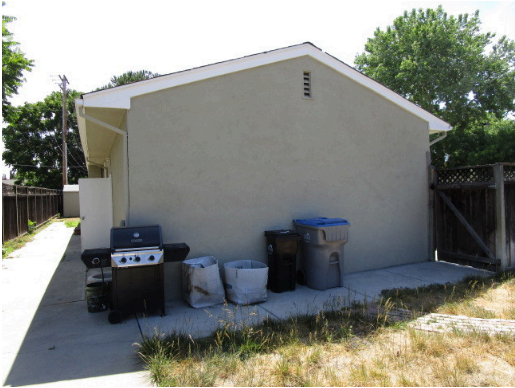
11. Western side of the 383 South Baywood Avenue residence
