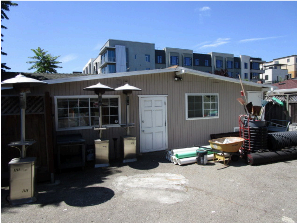
5. Northern side of the rear residential/storage building at the 375 South Baywood Avenue property
