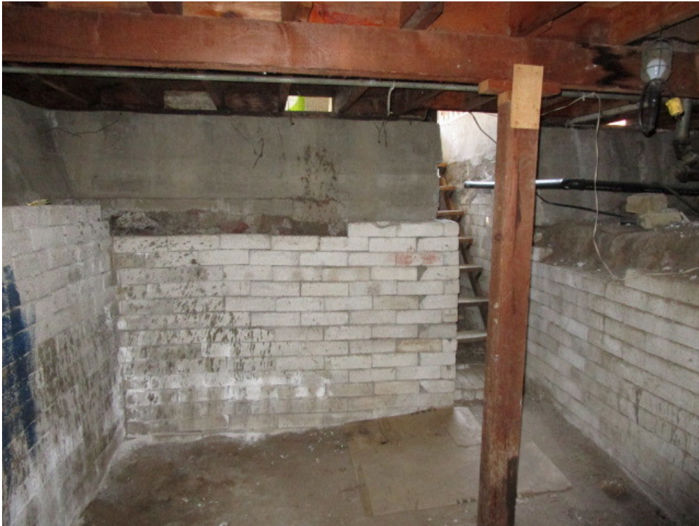
31. 376 South Baywood Avenue - partial basement
