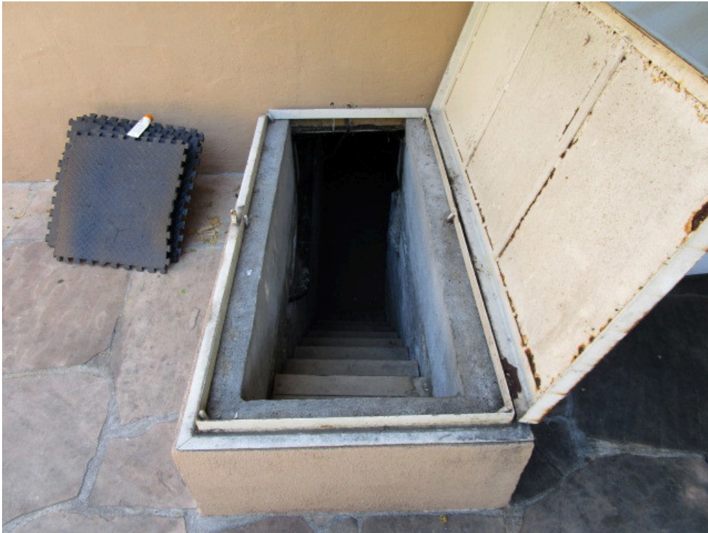
29. 376 South Baywood Avenue - entrance to partial basement
