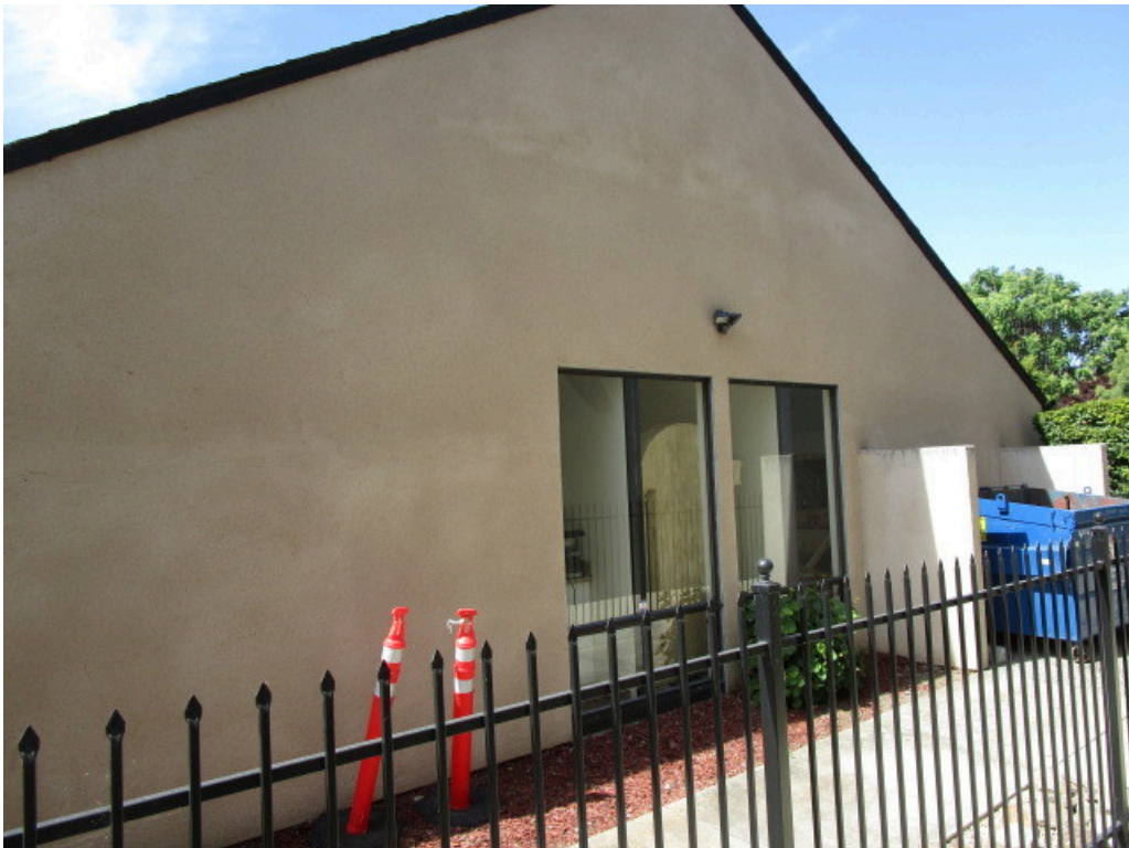
4. Northern side of the 2881 Hemlock Avenue building
