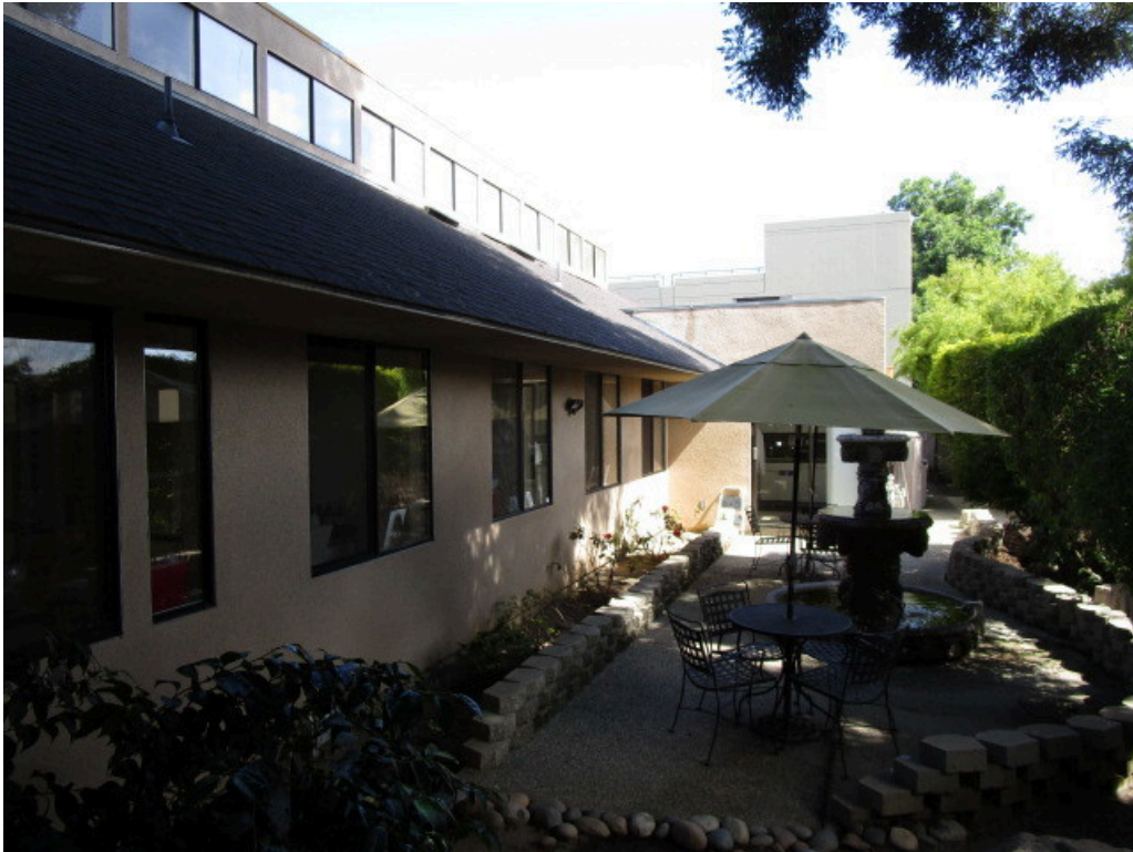
3. Eastern side of the 2881 Hemlock Avenue building
