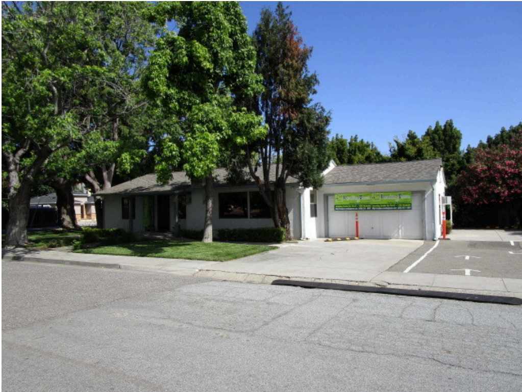
35. Ready Town (384 South Baywood Avenue) adjacent to the south and west
