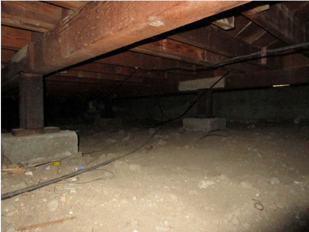
33. 376 South Baywood Avenue - crawl space
