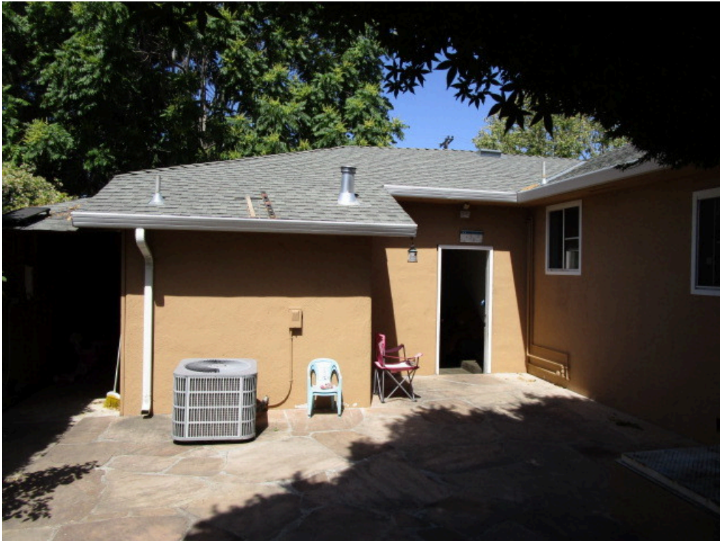
9. Eastern side of the 376 South Baywood Avenue residence
