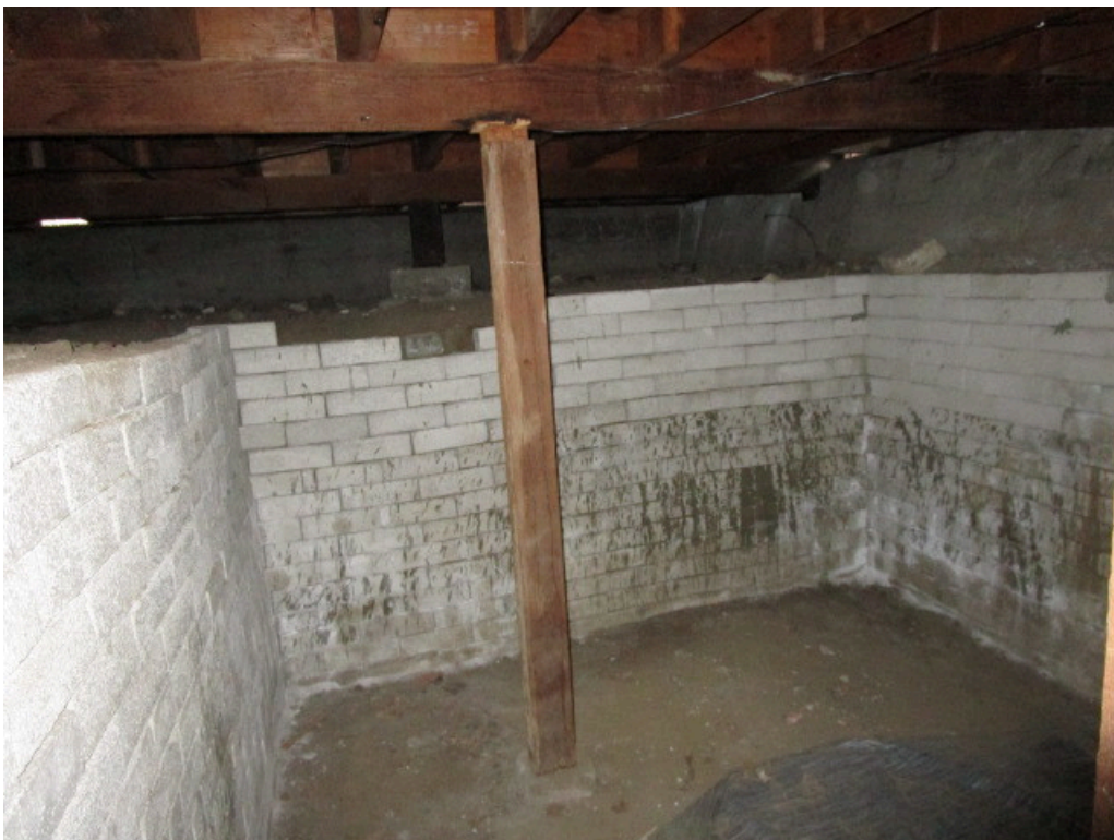
30. 376 South Baywood Avenue - partial basement
