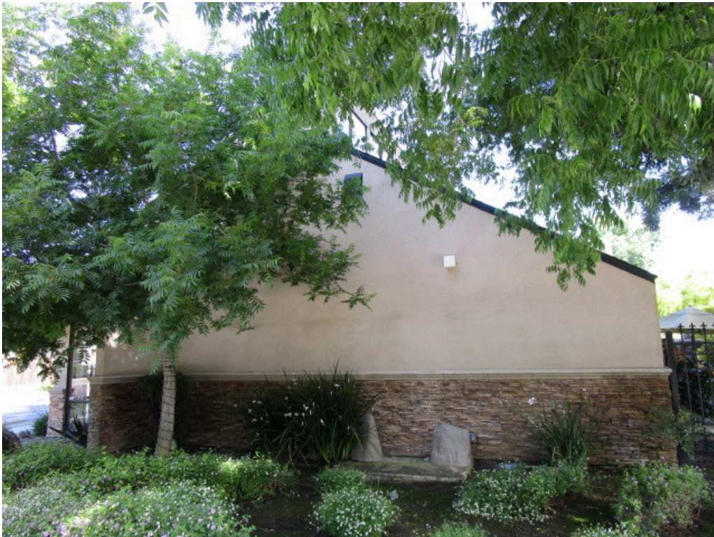
2. Southern side of the 2881 Hemlock Avenue building
