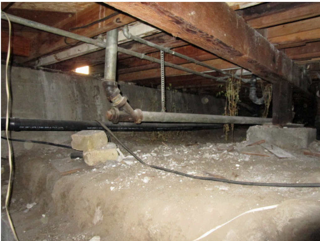
32. 376 South Baywood Avenue - crawl space
