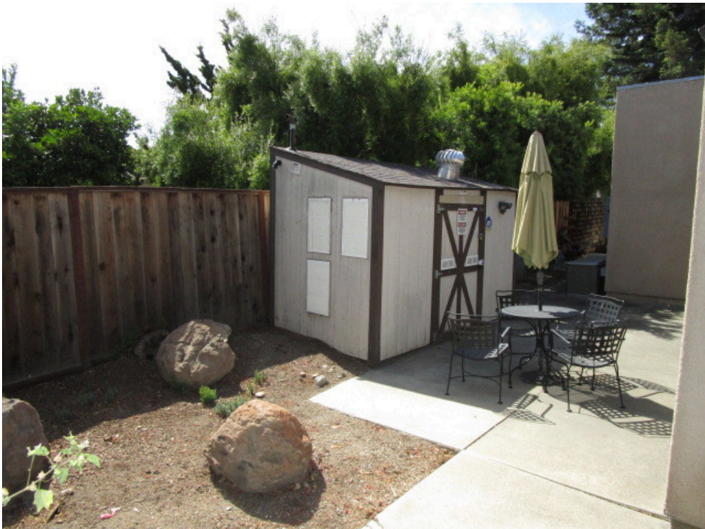
6. Compressor shed on the eastern side of the 2881 Hemlock Avenue building
