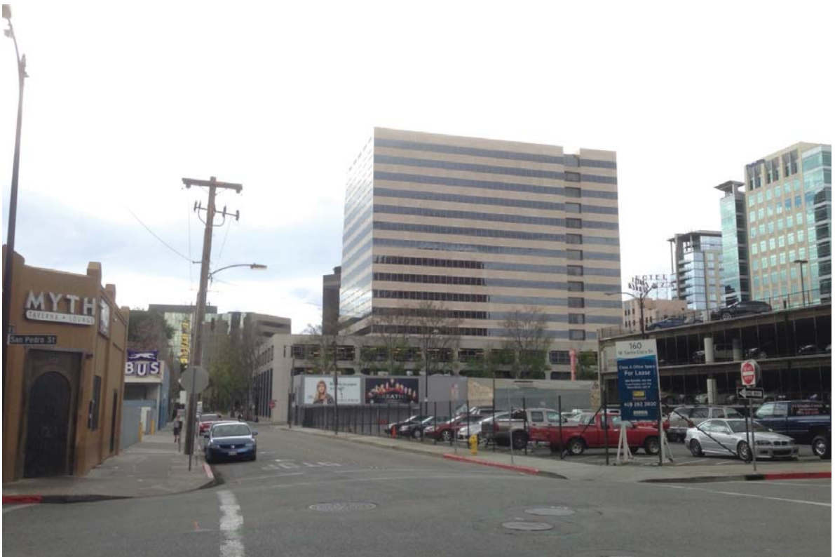
PHOTO 4: View of Post Street and the project site from the intersection of Post Street and S. San Pedro Street, looking northwest. The two billboards along the western site boundary are visible, as well as the surrounding low-to-high rise developments.
