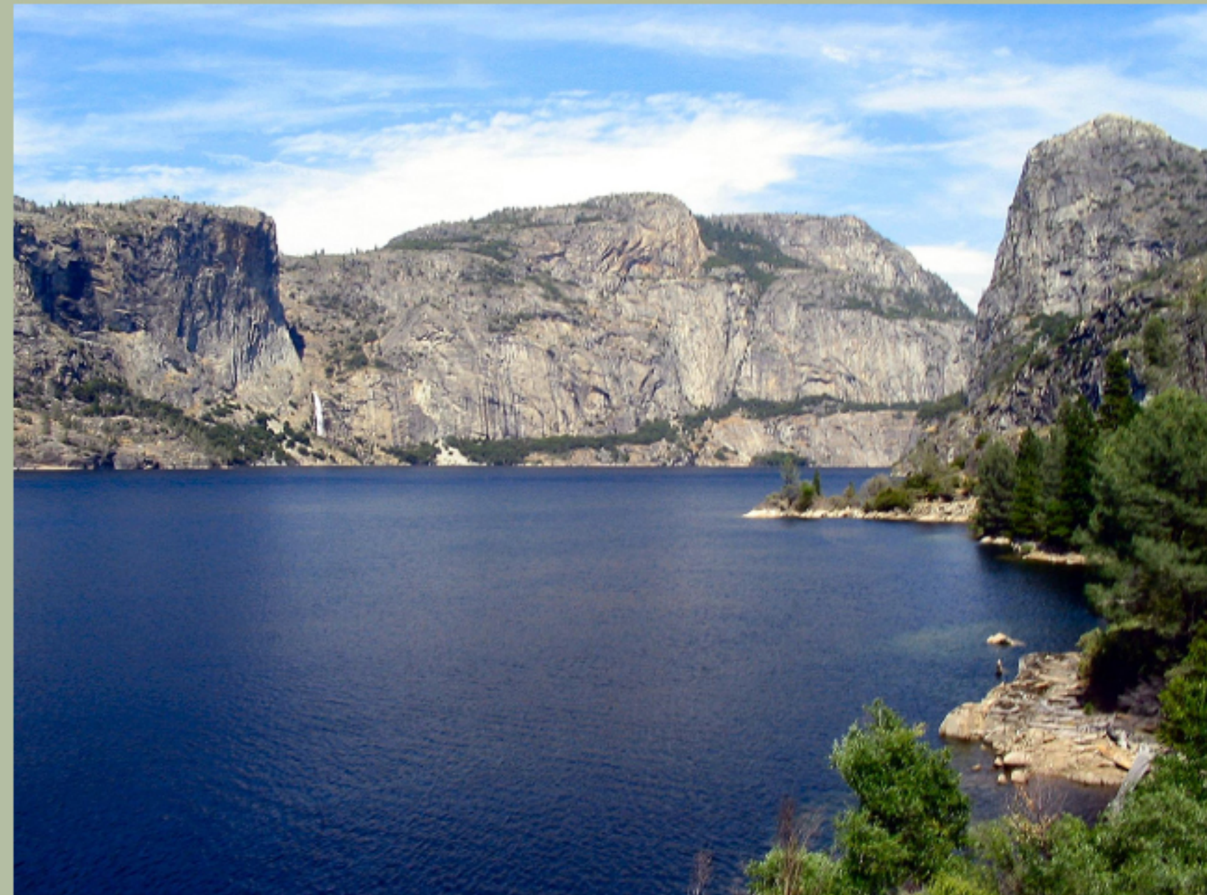
The Hetch Hetchy Reservoir in Yosemite National Park feeds Bay Division Pipelines No. 3 and 4, which run underground nearby
