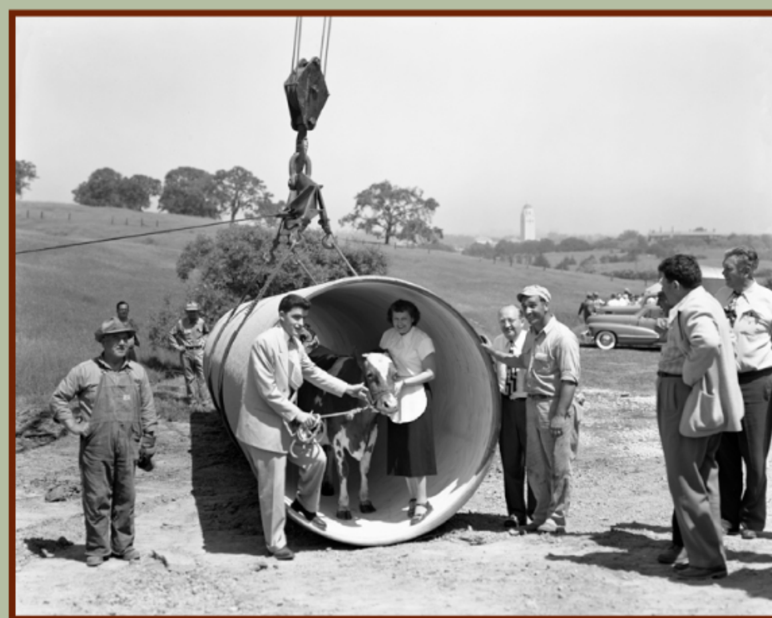
4/20/1950 — The laying of a 72-inch section of Bay Division Pipeline #3
