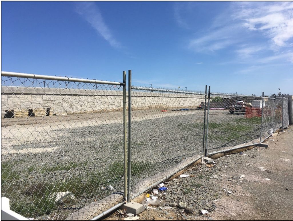
Photo 1: View of VTA Staging Site from northwest corner looking southeast.
