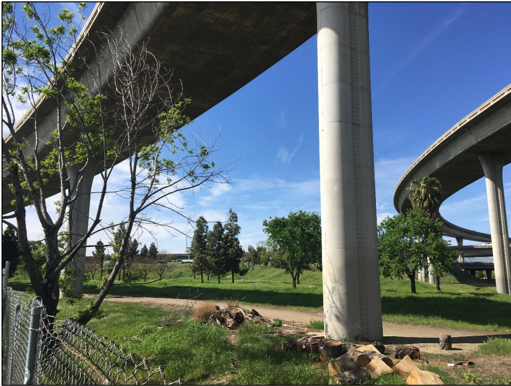
Photo 3: View of Felipe site from southwest corner looking north.
