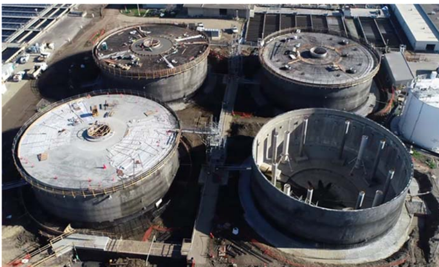
Figure 3: Roof replacement of Digesters 5-8 in various stages.
