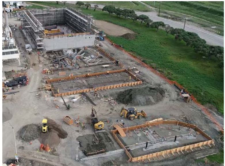
Figure 1: Cogeneration Facility Project concrete slab work continues
