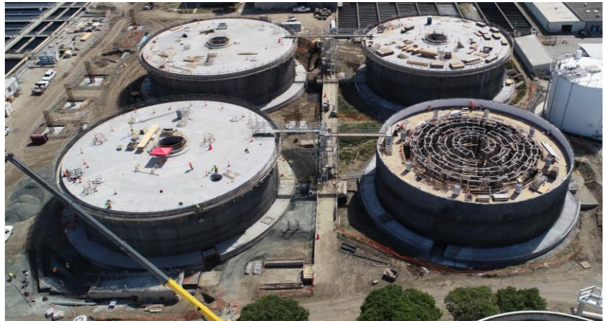
Figure 1: Digesters 5-8 showing ring beam construction
