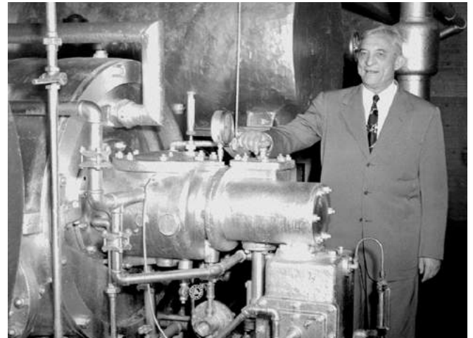
Figure 10: Willis Carrier (1922) proudly standing next to the first chiller. 61
