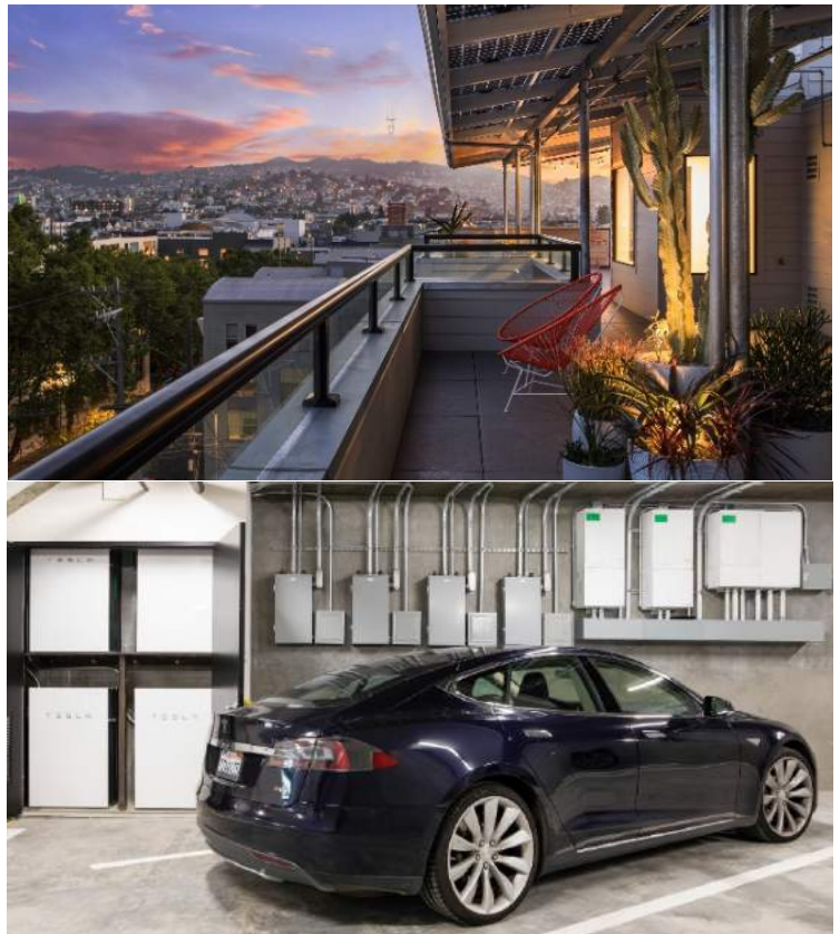
Figure 14: The Sol Lux Alpha apartment complex can operate as a “nanogrid” using the Tesla Powerwall 2, and vehicle to home charging.
