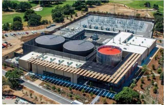
Figure 5. Stanford University's Central Energy Facility.
