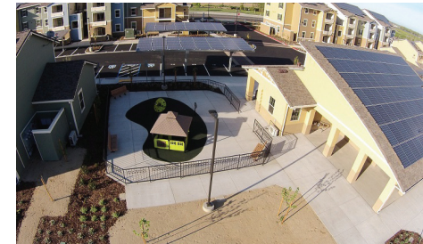
Spring Lake Apartments Woodland, CA Kuchman Architects Mutual Housing 2015 Frank Domin photo
