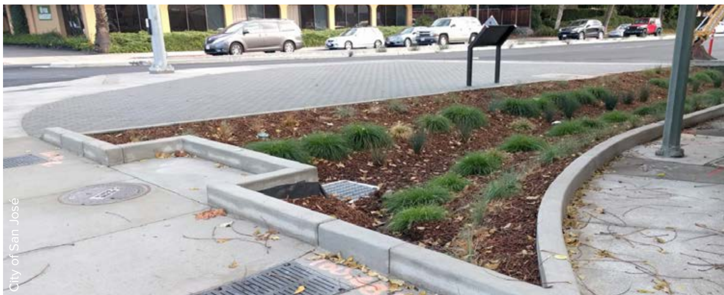
Green Street with Bioretention and Permeable Pavement on Park Avenue
