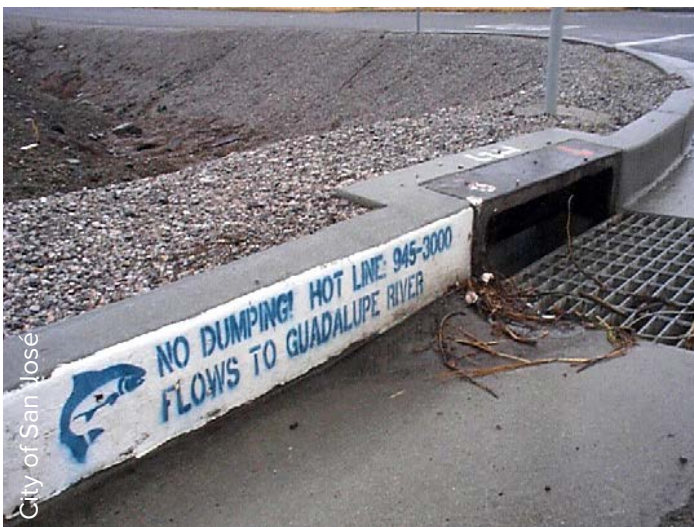
Storm Drain Draining to Guadalupe River
