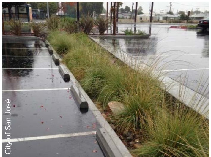
Bioretention in Commercial Parking Lot in San José
