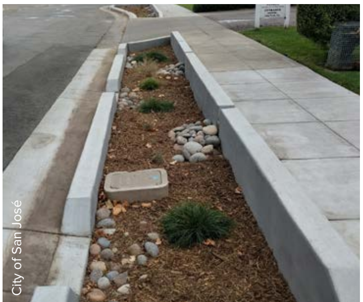
Figure 6-6. One of the Bioretention Areas Along Park Ave – Before and After
