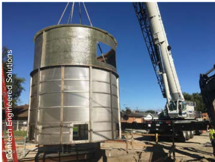
Installation of a Trash Capture Device in San José
