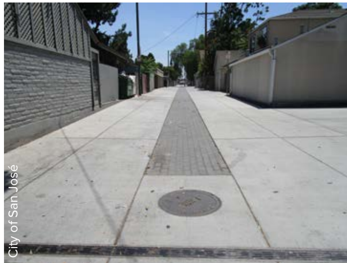
City of San José Permeable Pavement in Martha Gardens Alley Way
