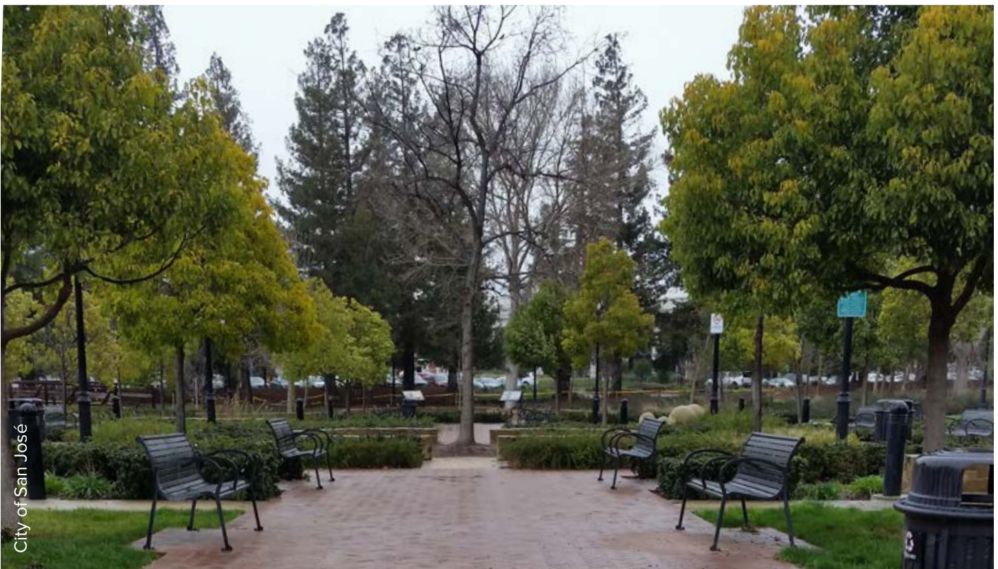
Permeable Pavement at Crescent Village Park in San José
