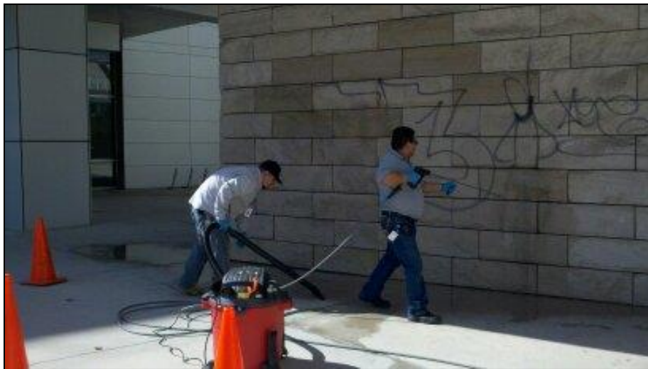
City of San José municipal staff use a shop vac during graffiti removal at City Hall.
