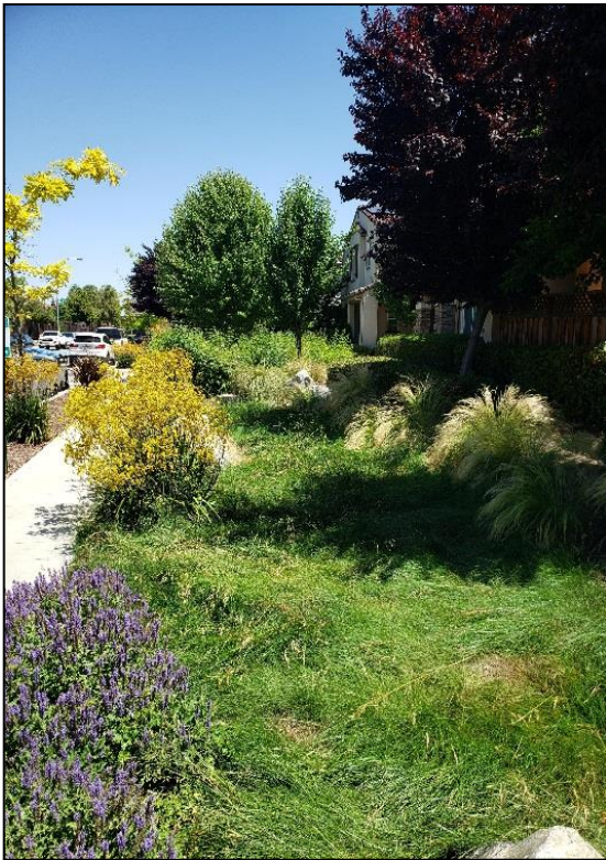
Bioretention installation in a residential area.
