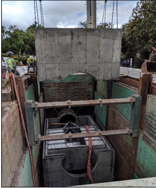
Installation of an HDS device at Rock Springs Drive.
