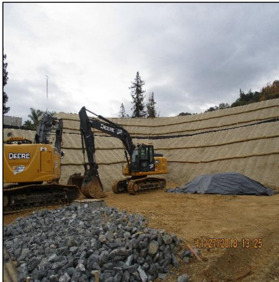
Effective BMPs installed on a hillside construction site.
