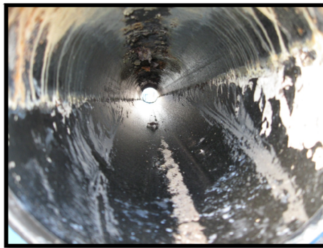
Figure 4-2. Heat exchanger that serves digester 5 showing no sign of scaling.
