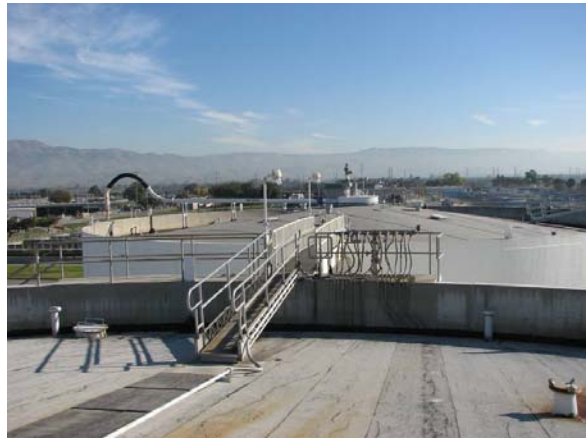
Figure 3-1. Existing San Jose WPCP digester floating covers
