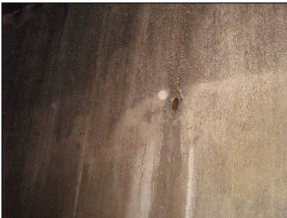
Photo 27. East wall in good condition, pipe penetration
