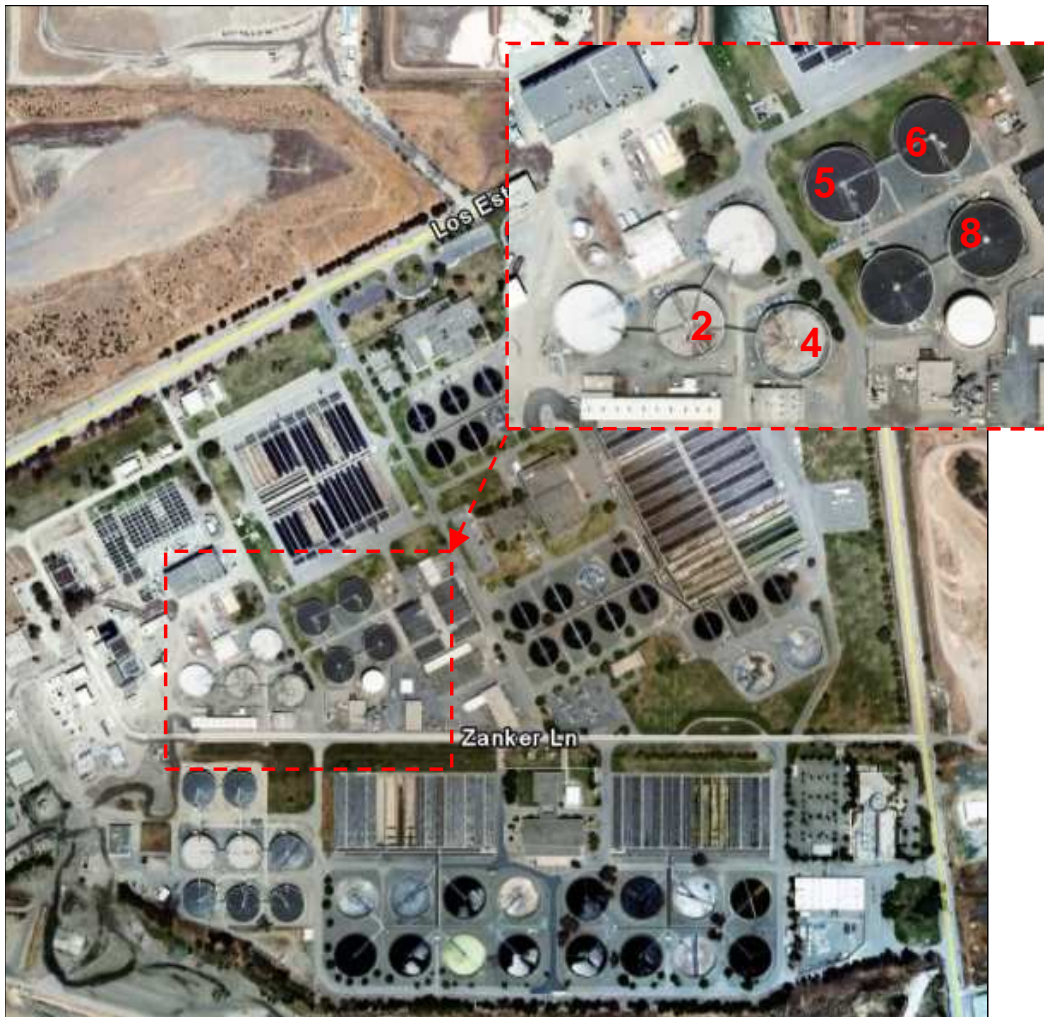
Figure 1.1 – San Jose Water Pollution Control Plant
