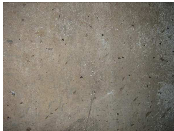
Photo 56. West wall in good condition (detail)
