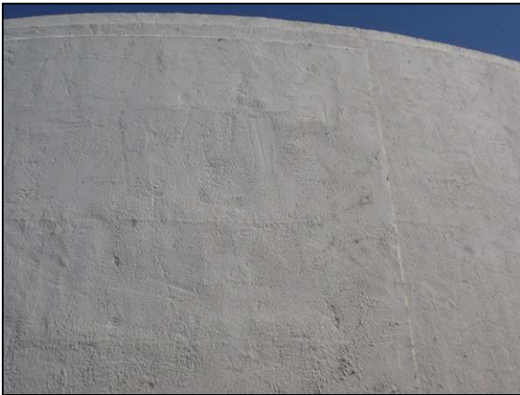
Photo 15. Exterior concrete wall in good condition
