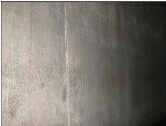
Photo 45. West wall in good condition
