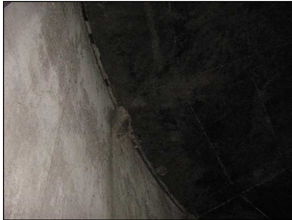
Photo 47. Steel interior roof in fair condition
