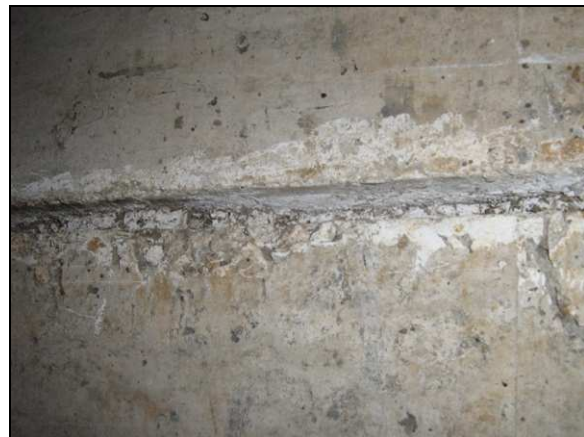
Photo 46. South wall joint in good condition
