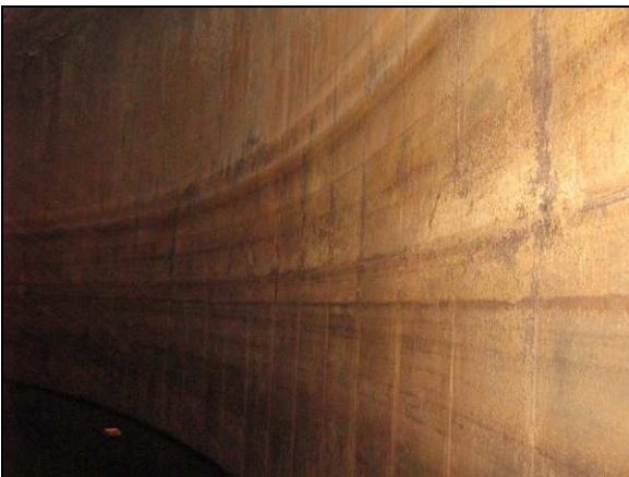
Photo 7. Interior wall in good condition
