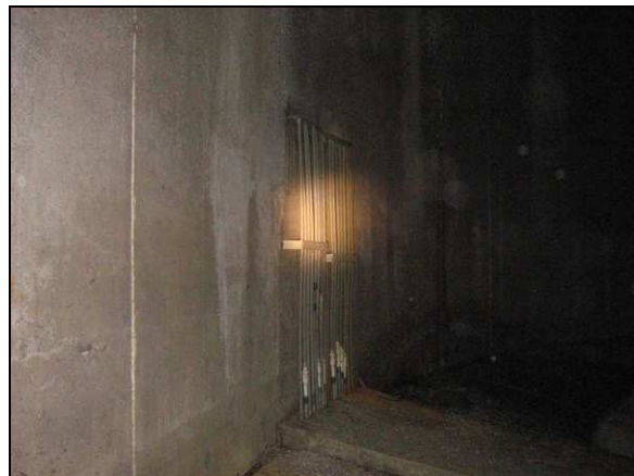
Photo 59. Conduits corroded on west wall in good condition
