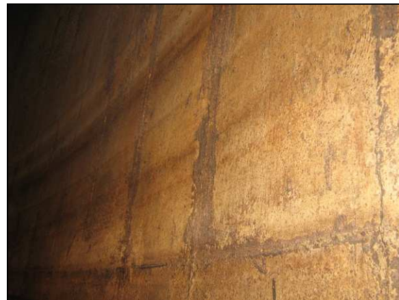
Photo 8. Interior wall (detail) in good condition
