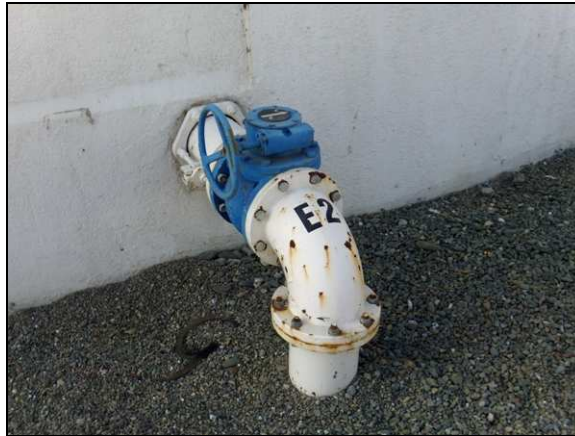
Photo 50. Minor corrosion staining on circulation pipe (typical)
