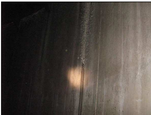
Photo 55. West wall in good condition
