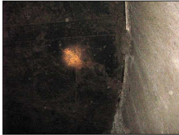
Photo 57. Steel interior roof in fair condition
