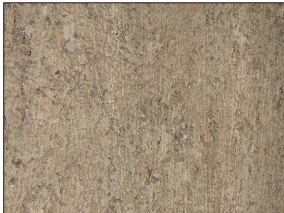
Photo 28. West wall (detail) in good condition
