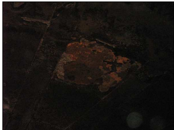
Photo 32. North roof with corroded area
