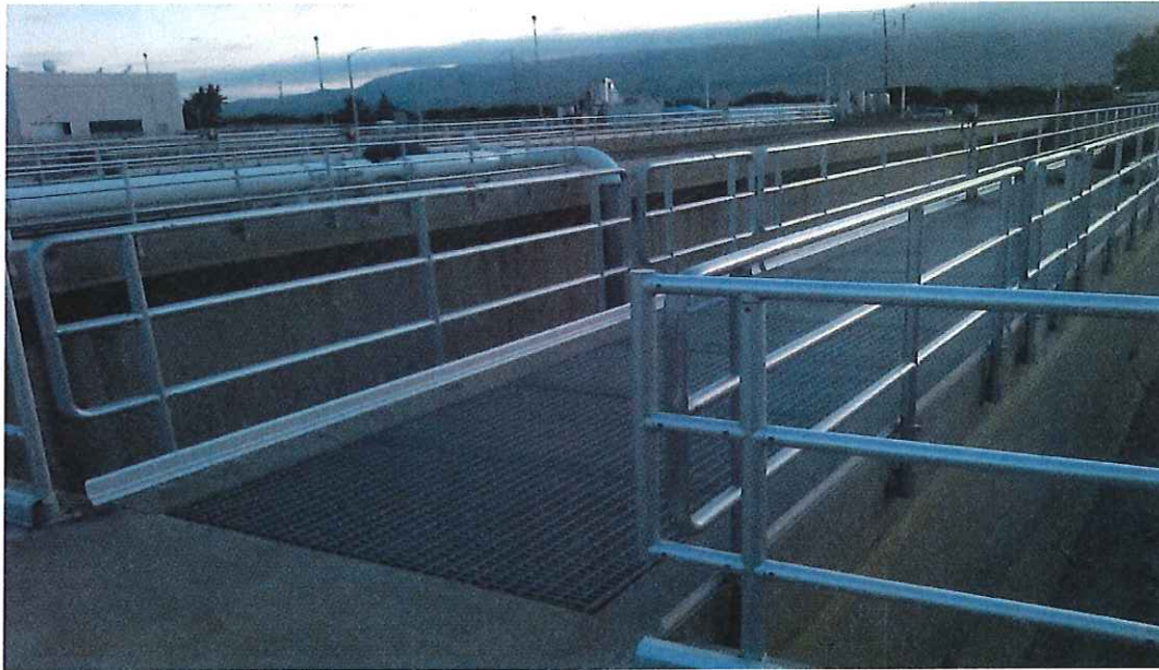
Figure 8— Handrail Replacement – Phase V
