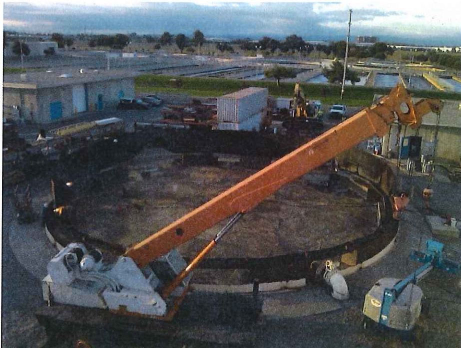
Figure 6—Digester Gas Storage Replacement, Demolition
