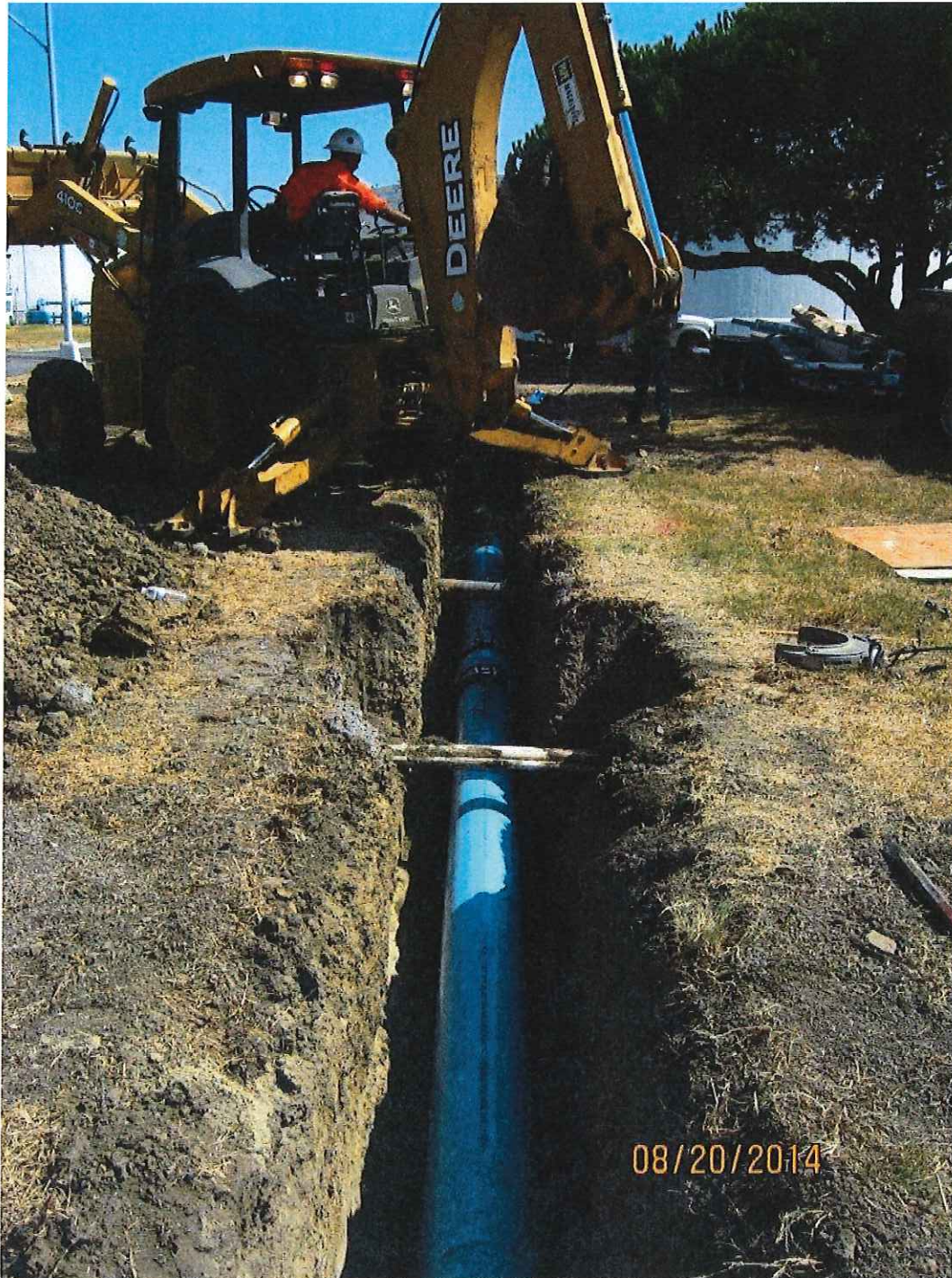
Figure 7— Fire Main Replacement - Phase III
