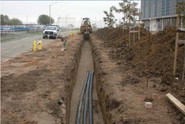
Fire main trench
