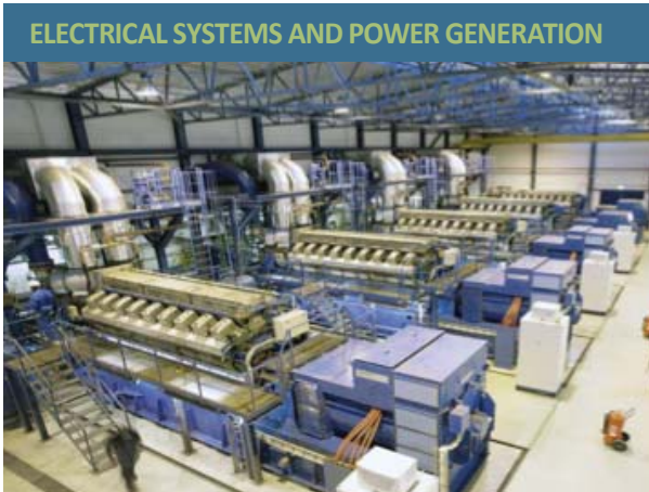
4 MW advanced internal combustion engines
